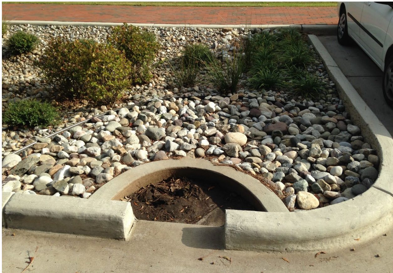
Figure 4: Example of Concrete-Lined Bioretention Forebay
