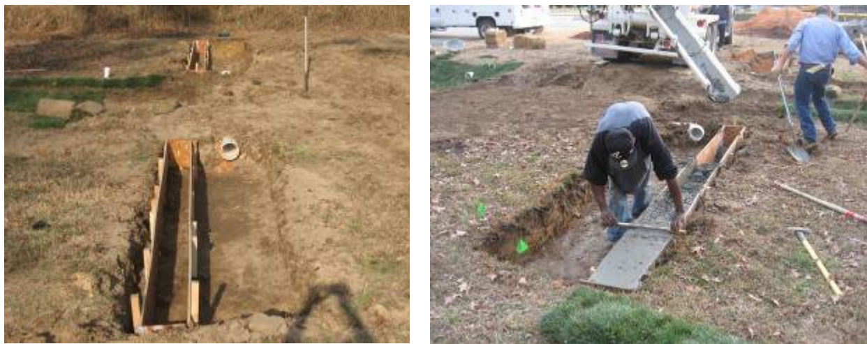
Figure 10: Forming the Level Lip (NCSU-BAE)
