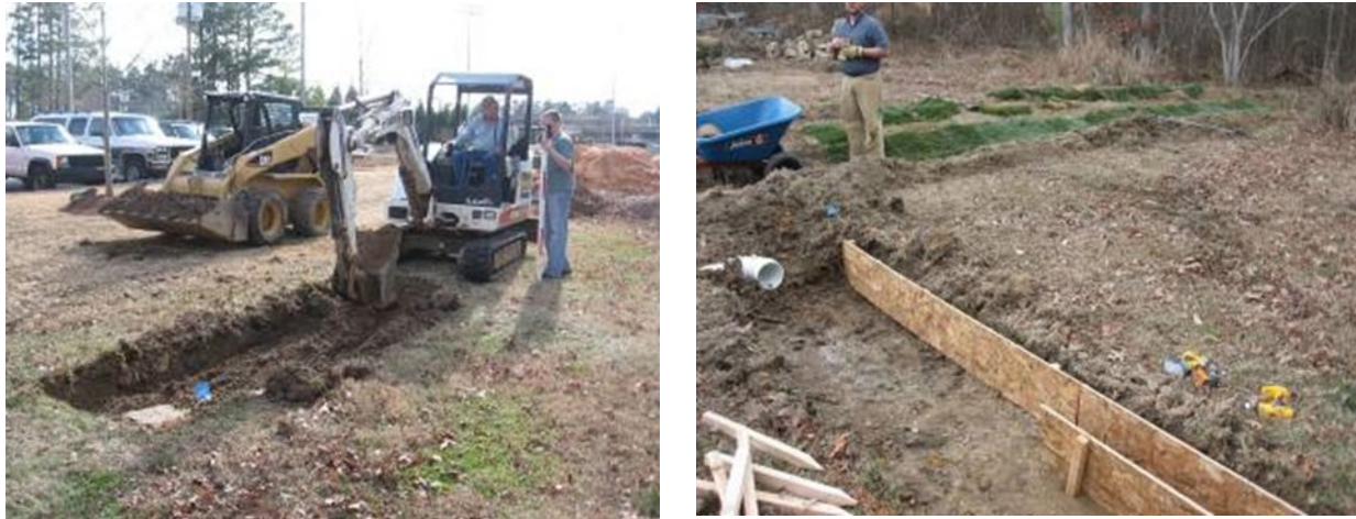
Figure 9: Excavating the Blind Swale (NCSU-BAE)
