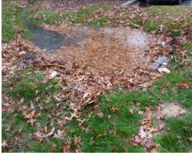
Figure 12: Clogged Forebay (left) and Unmaintained Blind Swale (right)
