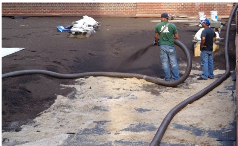
Figure 11. Growing media installation by crane hoist (left) and pneumatic blower (right) (Dr. Elizabeth Fassman)
