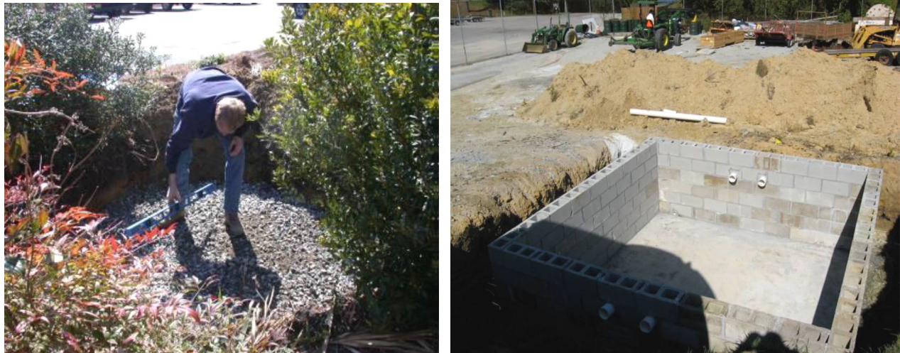
Figure 10. Preparing a cistern footing of aggregate (left) and a concrete footing for a cistern exceeding 1,500 gallons (right) (NCSU BAE)
