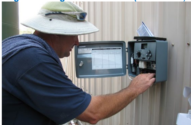
Figure 8. Irrigation Controller (NCSU BAE)
