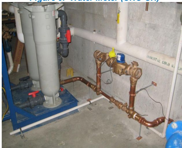
Figure 9. Water Meter (UNC-CH)
