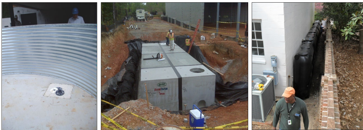
Figure 3. Metal cistern under construction (left), underground concrete vault wrapped in an impermeable liner (center) and a series of plastic cisterns (right) (UNC-CH left and NCSU BAE center and right)
