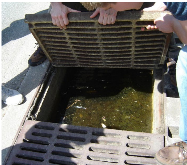
Clogged Sediment Chamber
