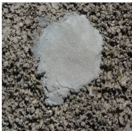
Figure 19. Pavement Patch
