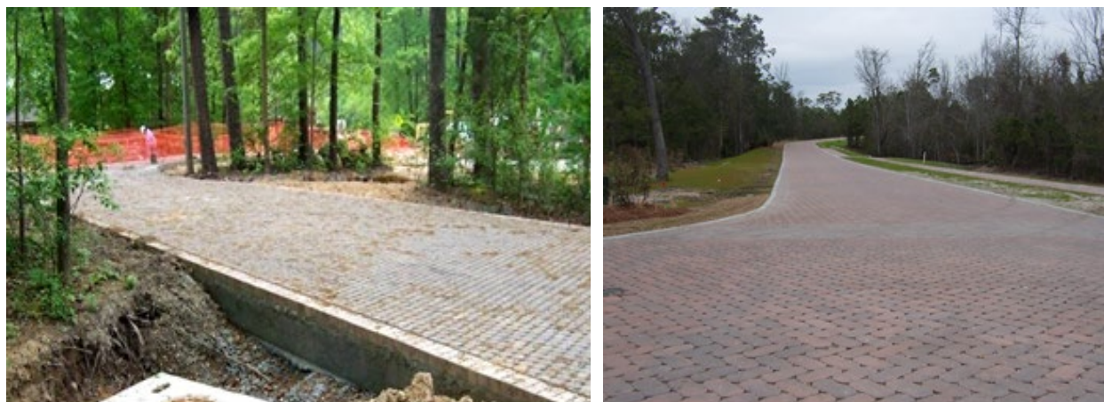
Figure 5. Edge Restraints on PICP
