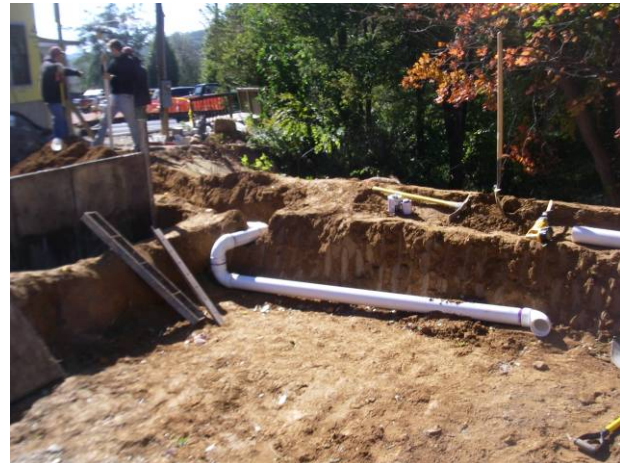
Figure 11. Upturned Elbow (NCSU-BAE)
