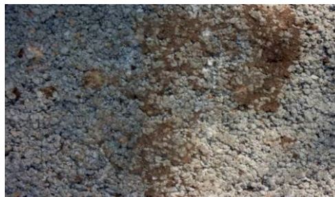
Figure 15. Clogged Pavement
