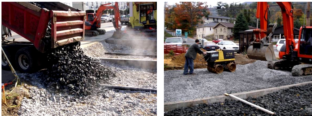
Figure 12. Aggregate Placement and Compaction (NCSU-BAE)
