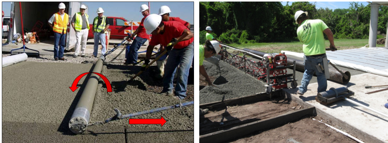
Figure 14. Compacting Pervious Concrete (NCSU-BAE)
