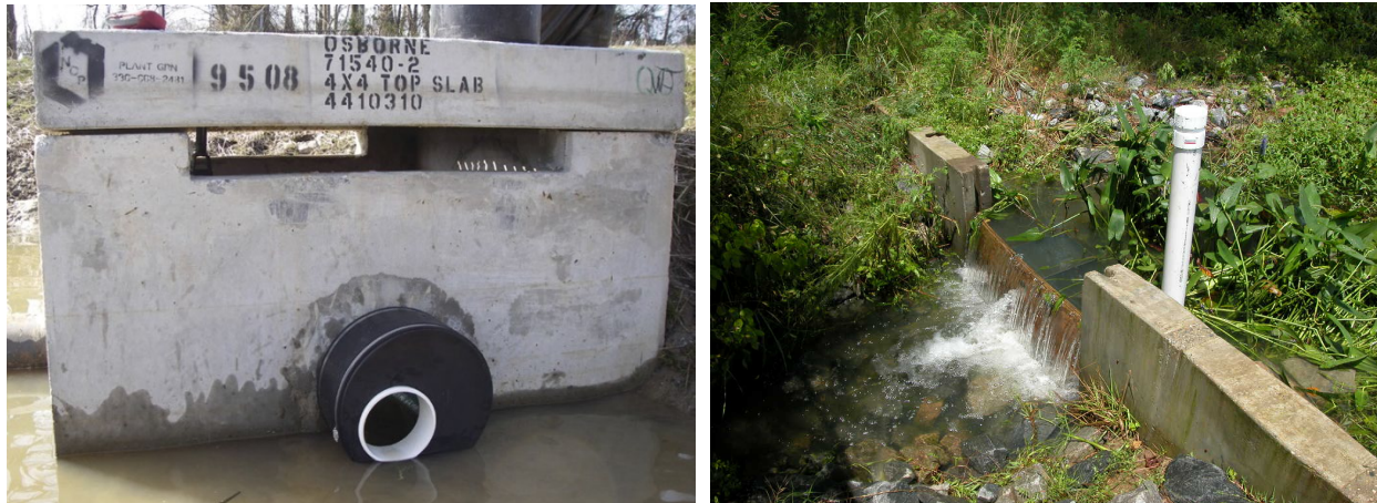
Figure 4: Two Examples of Adjustable Outlets
