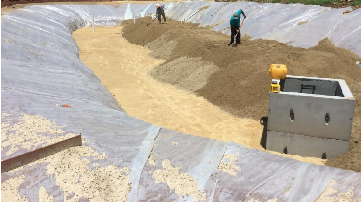
Figure 2: Covered Side Slopes to Protect Bioretention Media During Construction
