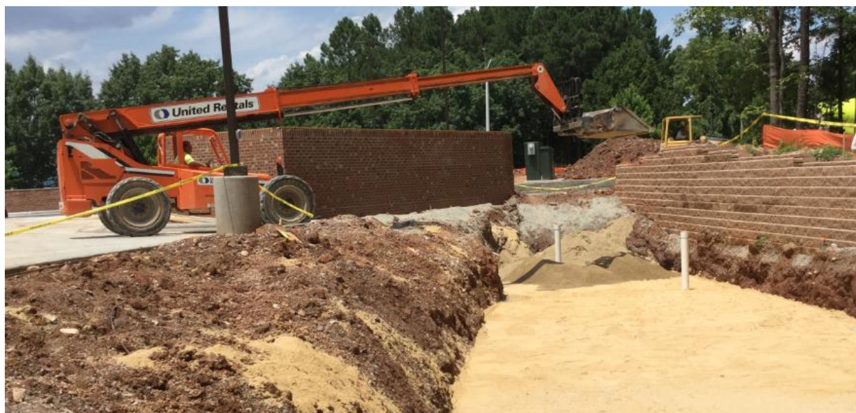
Figure 1: Using Proper Equipment to Avoid Media Compaction During Construction
