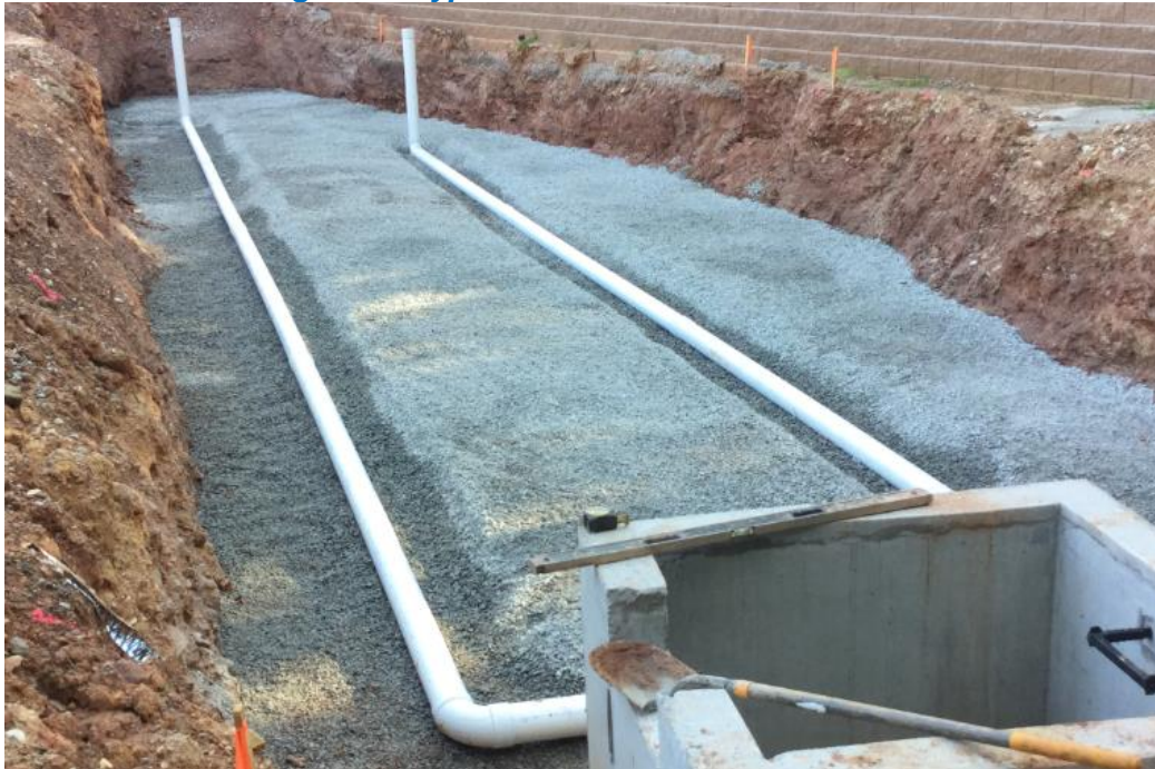
Figure 4: Typical Bioretention Underdrain
