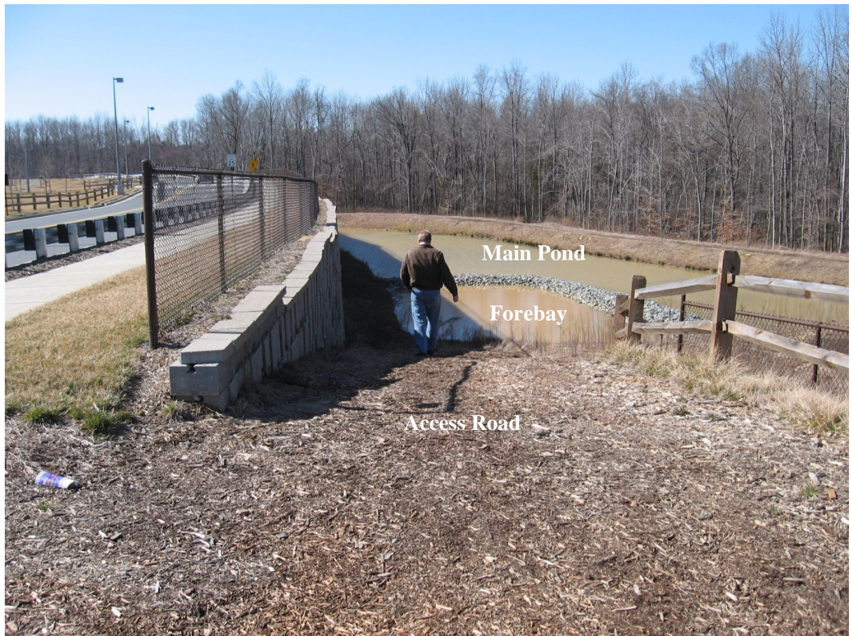
Figure 4.3 Maintenance Access Road
