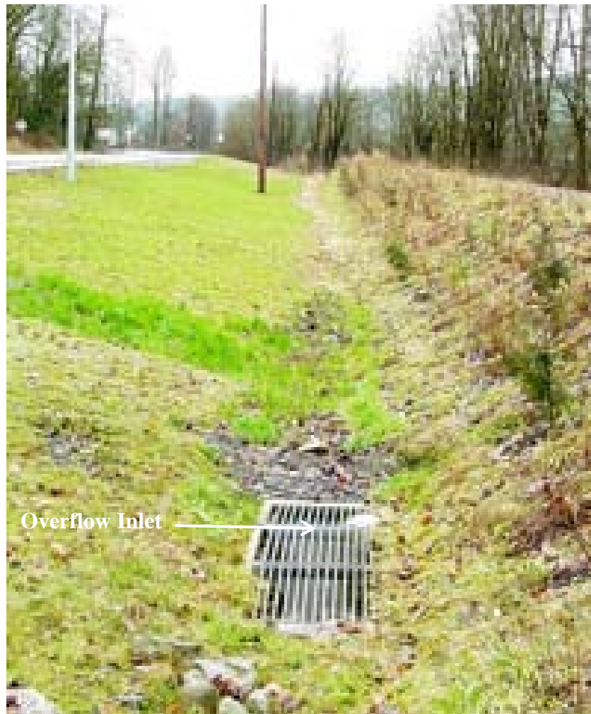
Figure 7.1 Filter Strip Inlet
