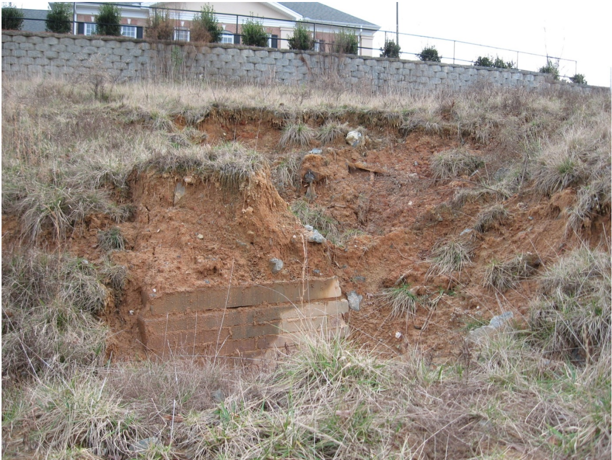
Figure 4.10 Embankment Erosion
