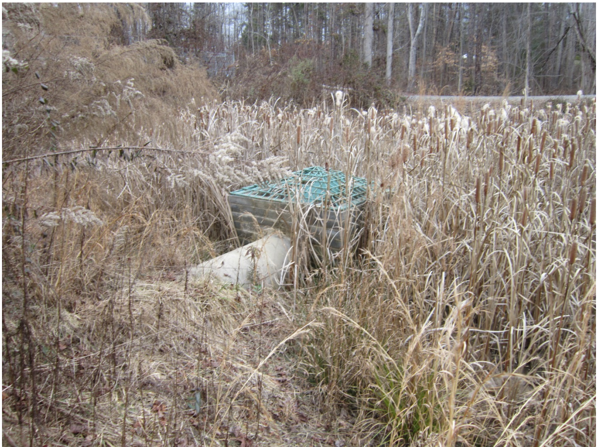
Figure 8.3 Over Grown Dry Detention
