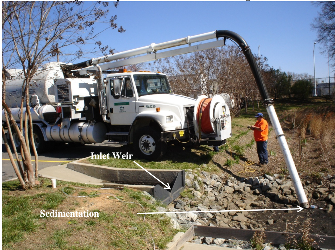
Figure 3.4 Forebay Vacuuming
