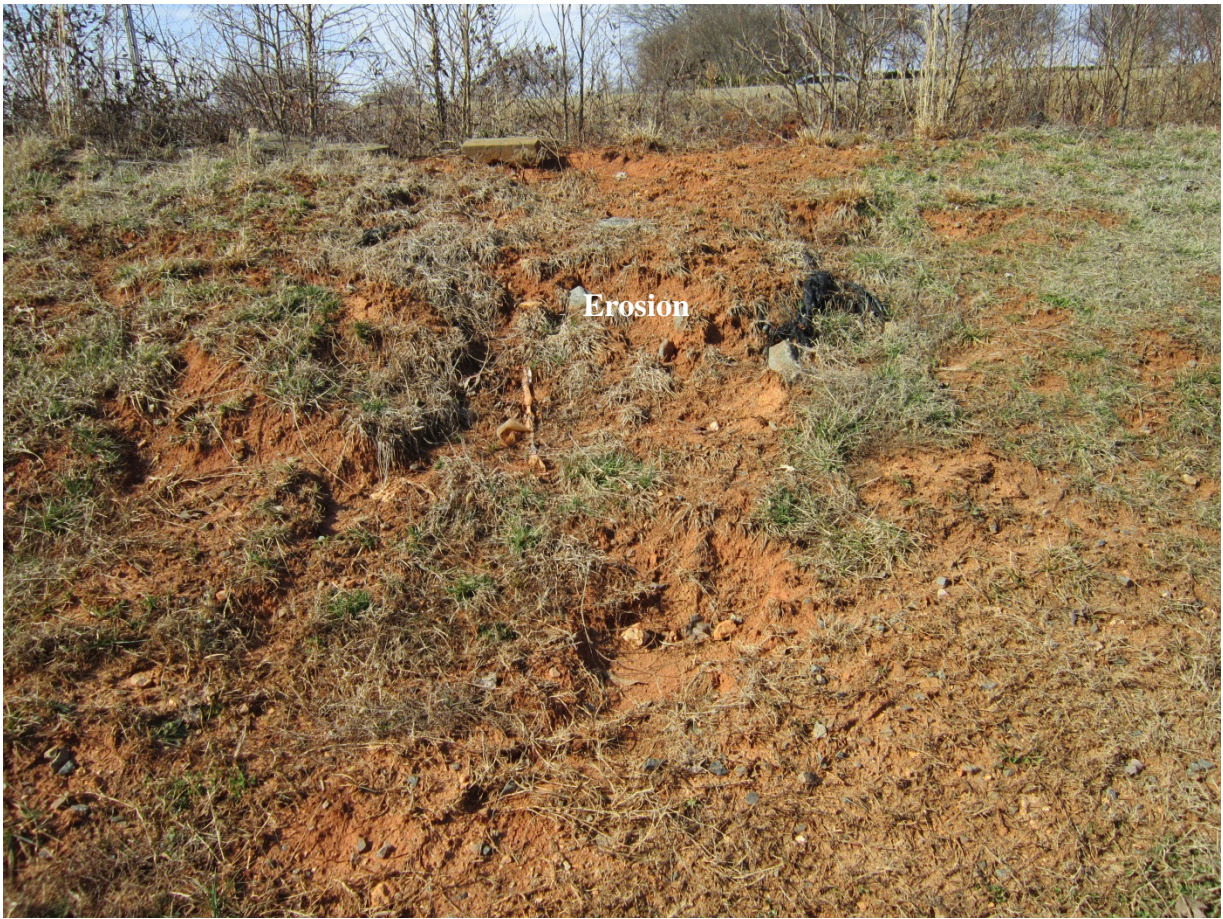
Figure 4.13 Slope Erosion
