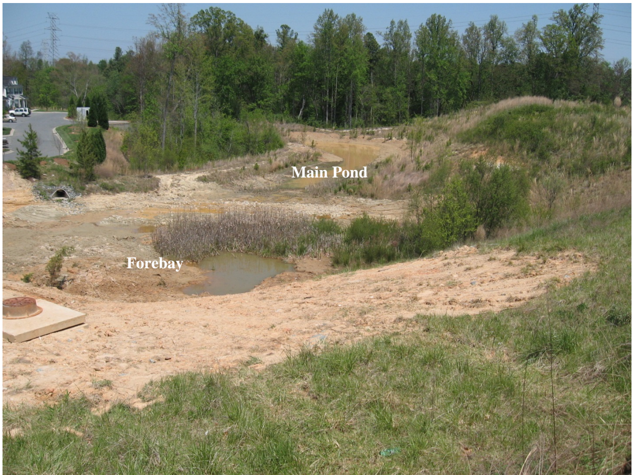
Figure 4.8 Wetpond Excavation
