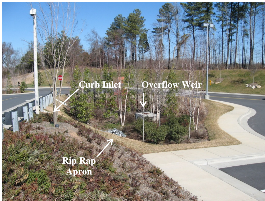
Figure 3.1 Well-maintained Bioretention Facility
