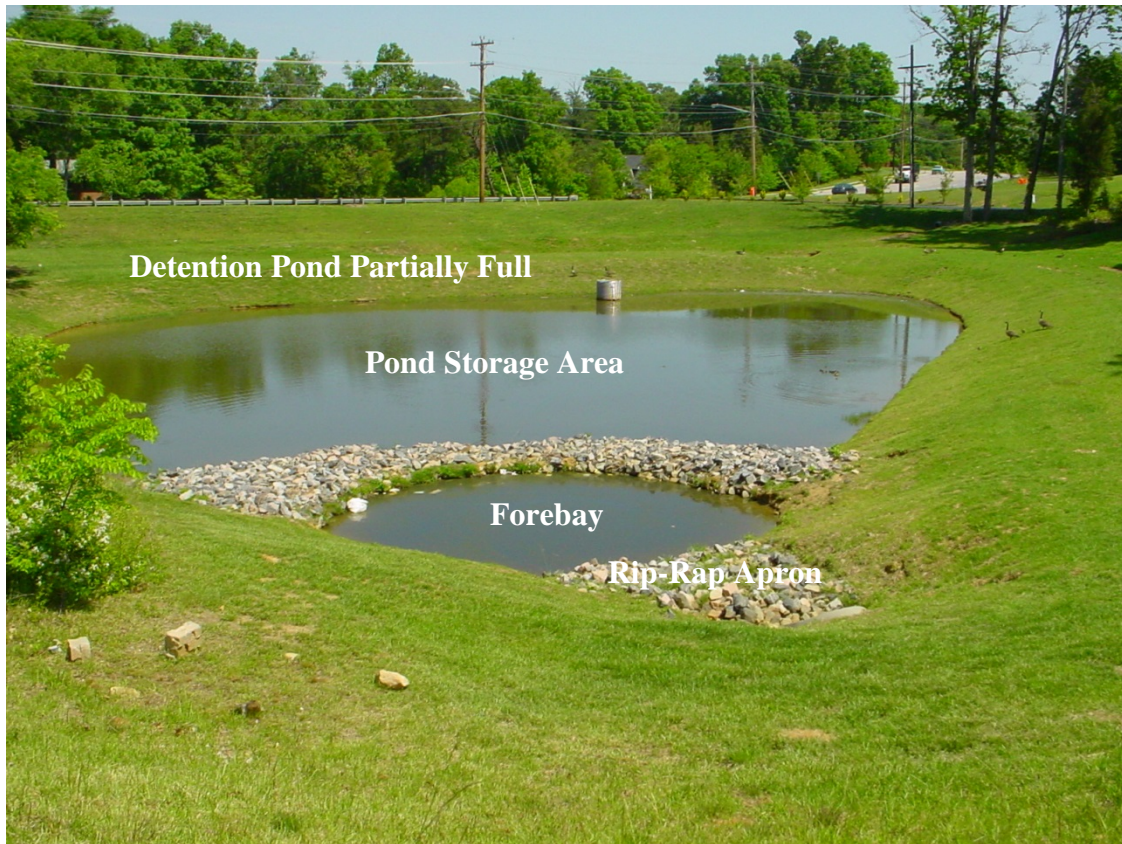
Figure 8.1 Partially Full Dry Detention Basin
