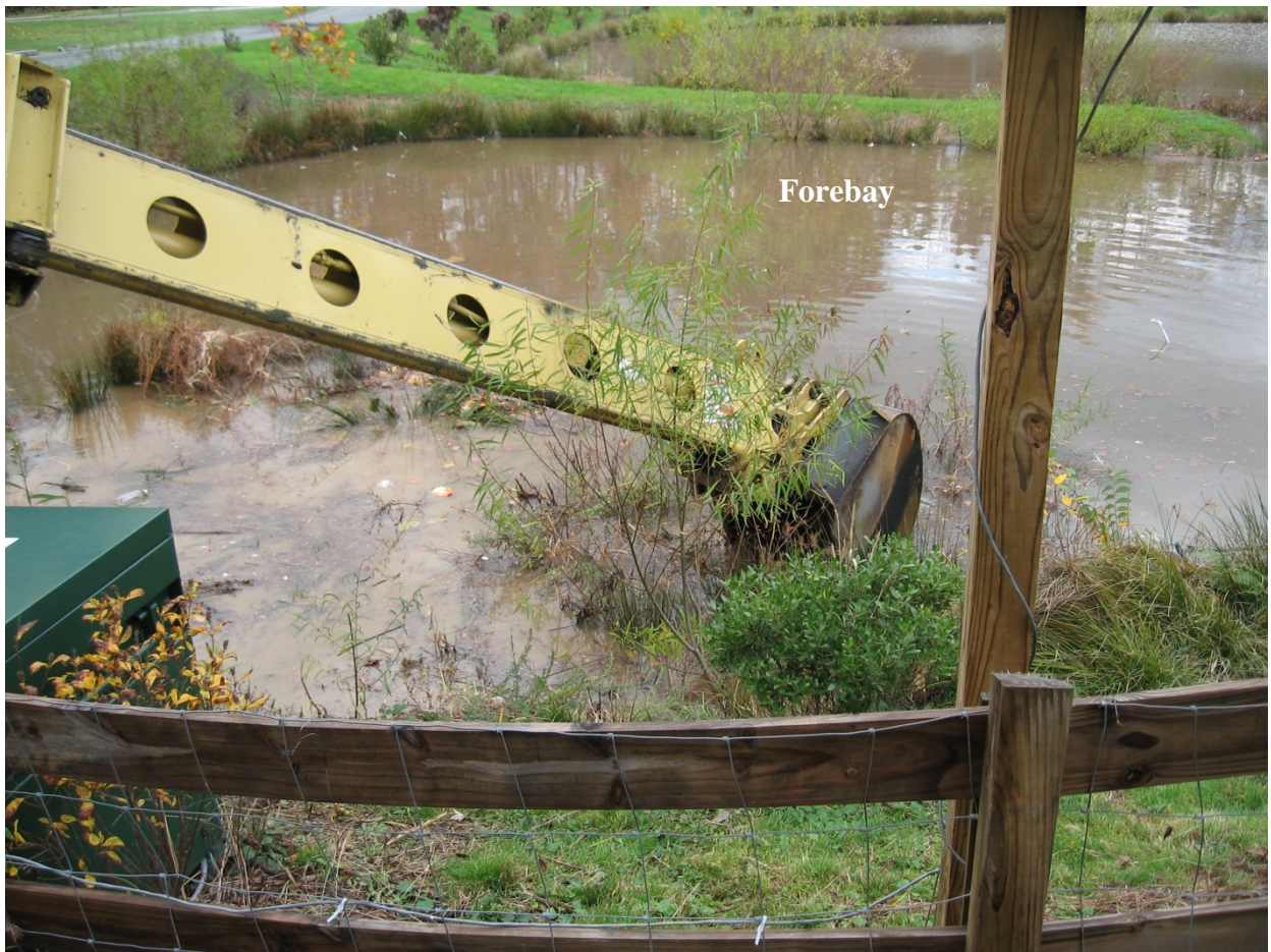
Figure 4.5 Excavating Forebay
