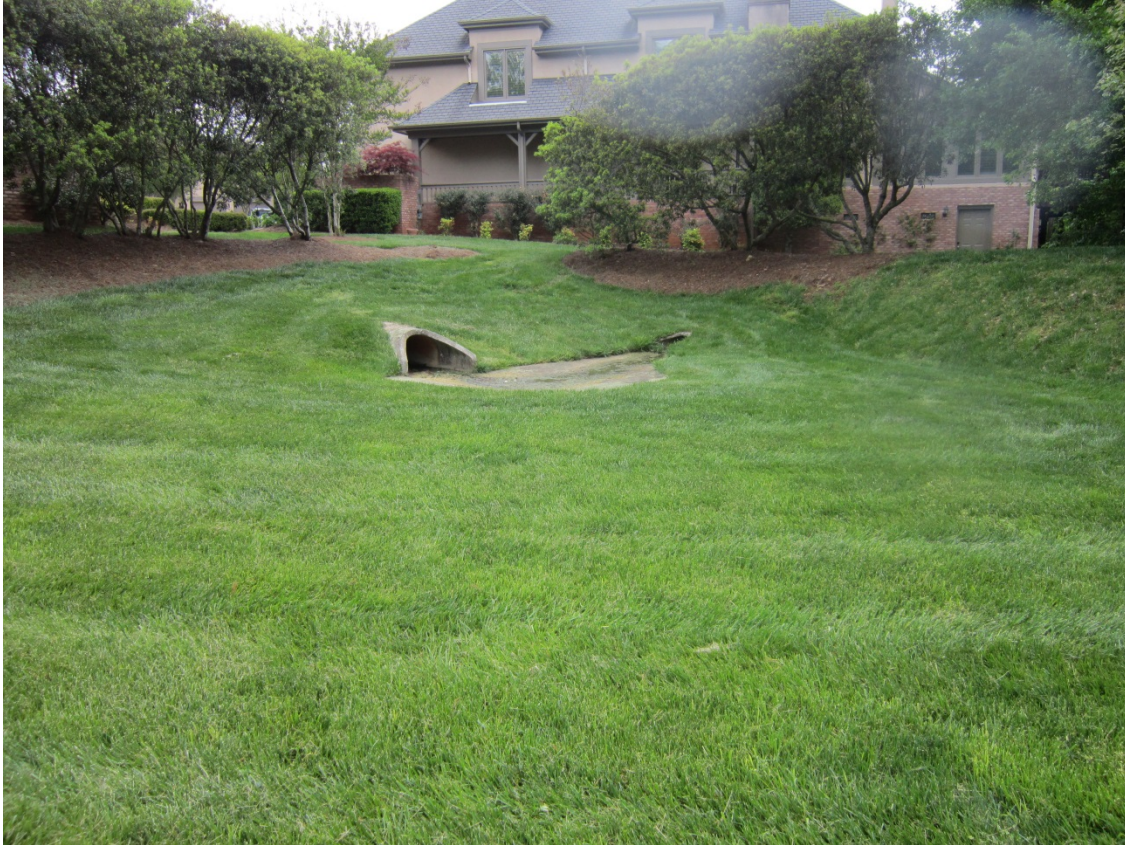
Figure 8.2 Well Maintained Detention Basin
