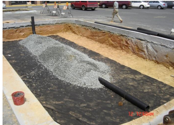
Figure 4: Installation of Under Drain
