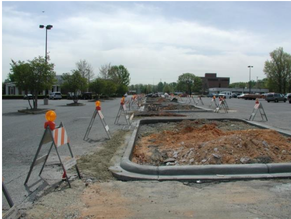
Figure 3: Installation of Curbing
