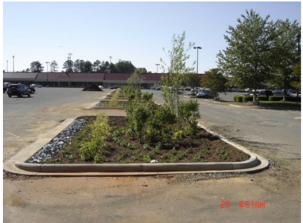
Figure 6: Installation of Mulch and Plantings
