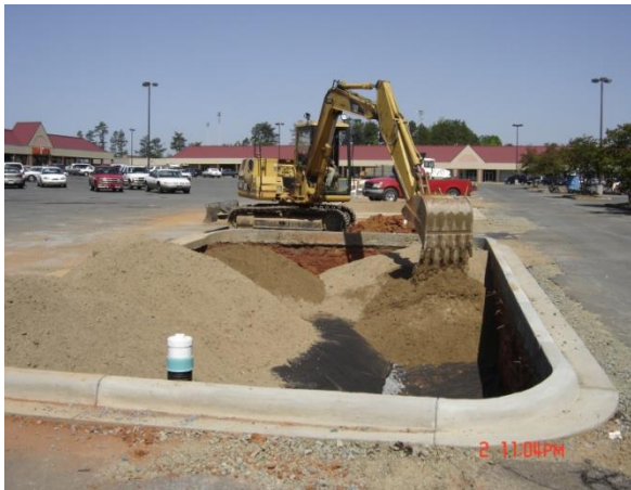
Figure 5: Installation of Bio Soil Media
