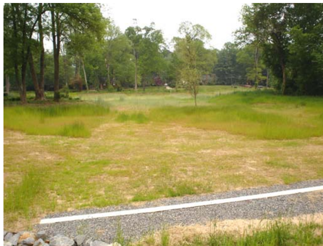
Figure 1: Filter strip down slope of level spreader.
