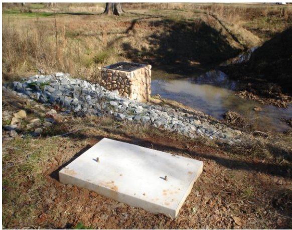
Figure 5: Outlet riser and monitoring box pad
