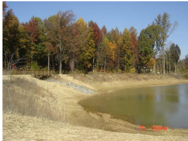
Figure 6: Installation of final bank seeding
