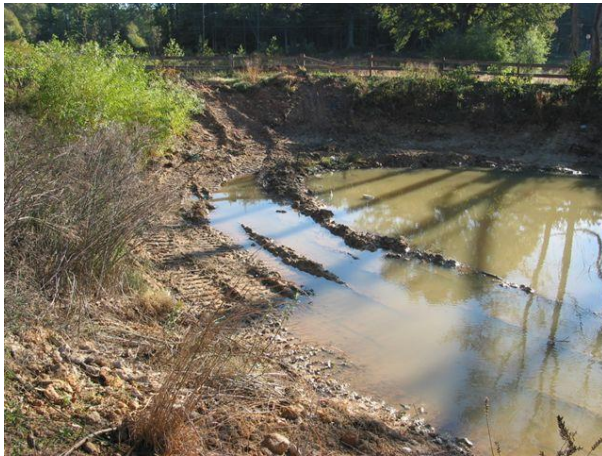
Figure 5: Littoral shelf grading
