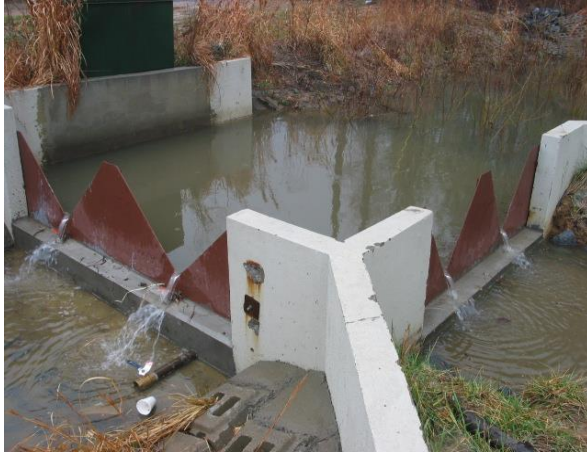
Figure 7: Inlet weir and flow splitter
