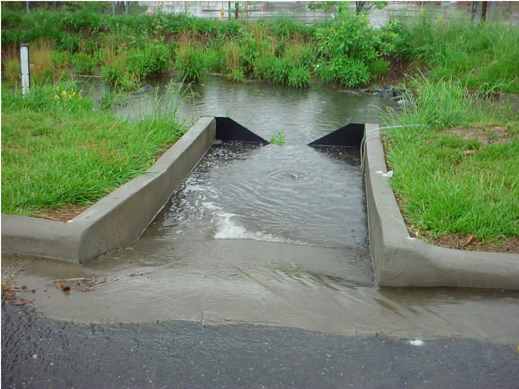
Figure 2. 120° weir at the HMBC inlet.
