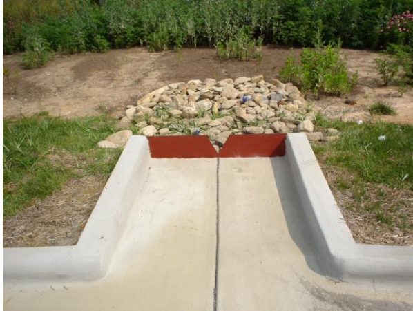
Figure 7: Bioretention inlet monitoring weir
