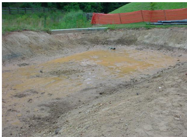
Figure 3: Basin excavation
