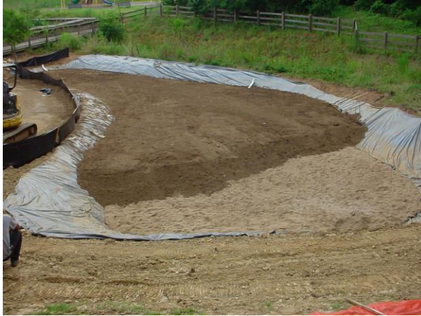
Figure 5: Installation of sand & bio soil media layers
