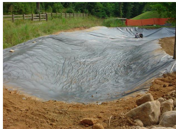
Figure 4: Sub-surface PVC liner installation
