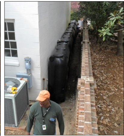
Figure 3. Metal cistern under construction (left), underground concrete vault wrapped in an impermeable liner (center) and a series of plastic cisterns (right) (UNC-CH left and NCSU BAE center and right)
