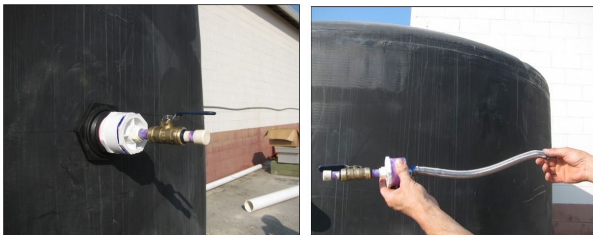
Figure 5. Anti-Clogging Passive Drawdown Mechanism (NCSU BAE)
