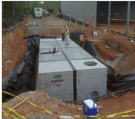
Figure 3. Metal cistern under construction (left), underground concrete vault wrapped in an impermeable liner (center) and a series of plastic cisterns (right) (UNC-CH left and NCSU BAE center and right)
