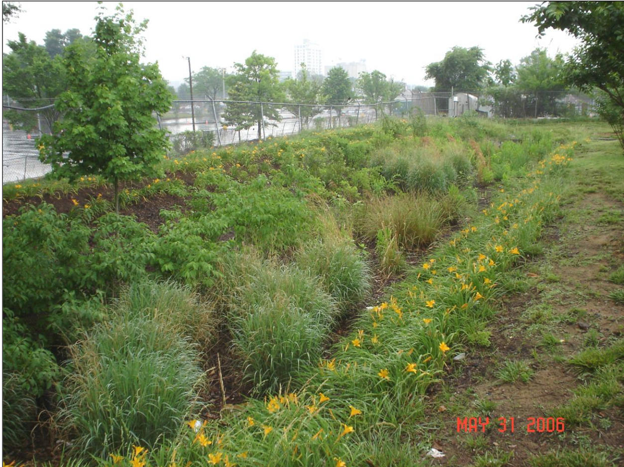
Figure 8.3. Planted and Mulched Rain Garden
