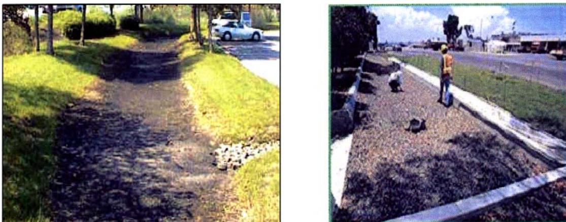
Figure 4.6.1 Examples of Infiltration Trench BMPs
