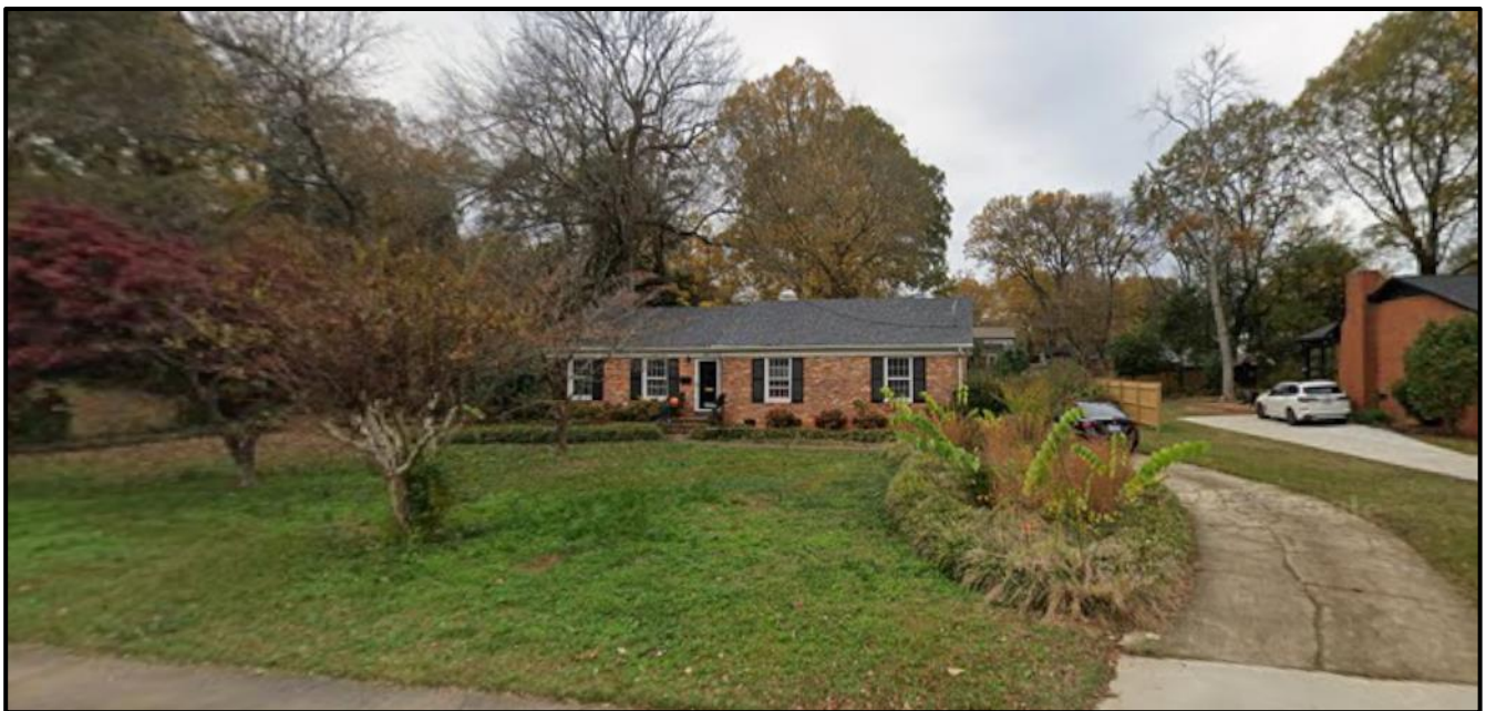
The site viewed from Murrayhill Road.
