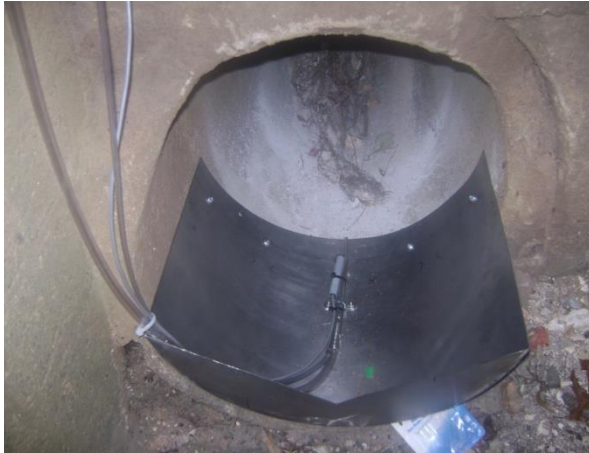
Figure 4: In-Line Monitoring Weir
