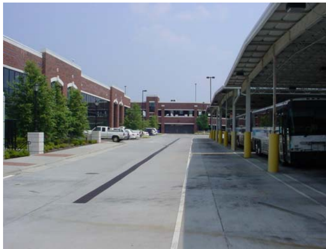
Figure 1: Photo of watershed area draining to BMP
