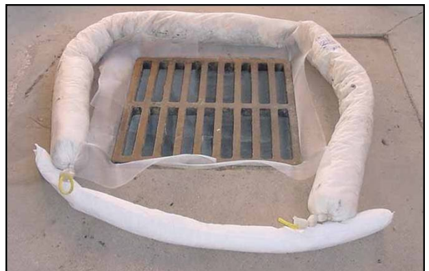
Oil absorbent socks and mesh screen can be effective at filtering pollutants.
