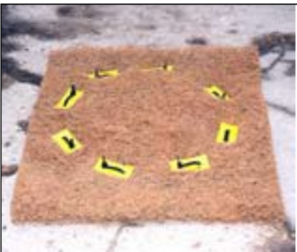
A natural fiber drain cover/filter that attaches to the top of a storm drain catch basin.
