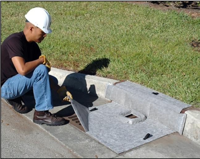
This type covers the entire drain entrance and attaches without removing the grate.
