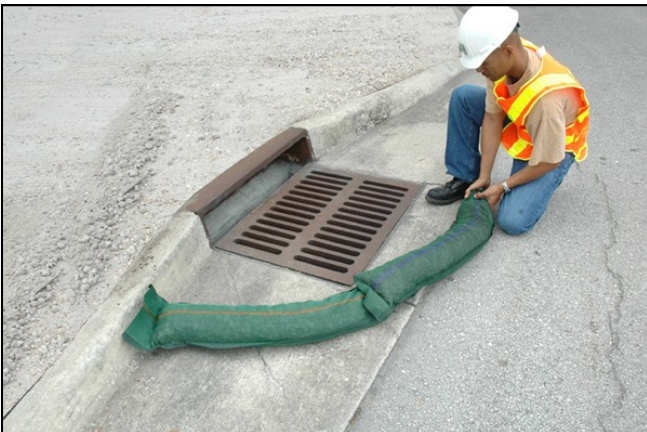
Rock-filled bags placed around a storm drain will filter pollutants.
