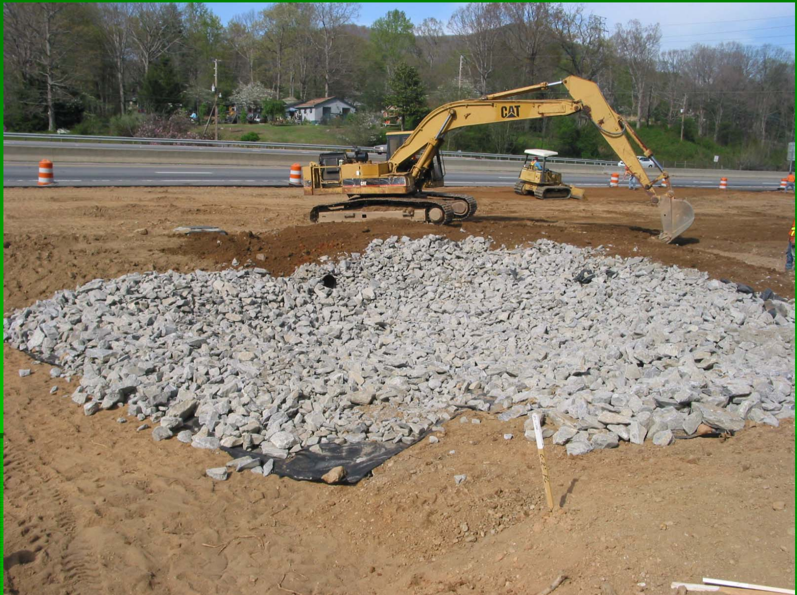
Placement of Rip Rap in sediment forebay
