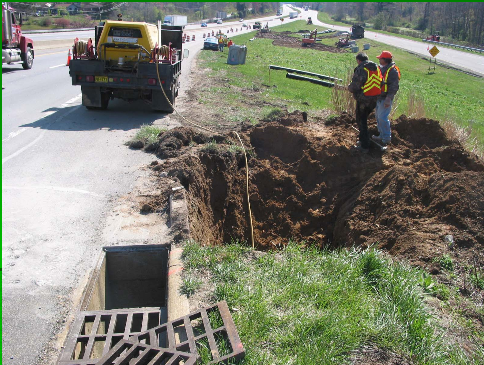
Preparation for drilling into upper existing drop inlet at end of bridge deck
