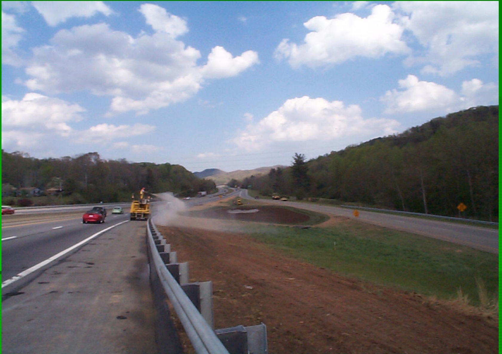
Hydro seeding disturbed areas outside of sod perimeter
