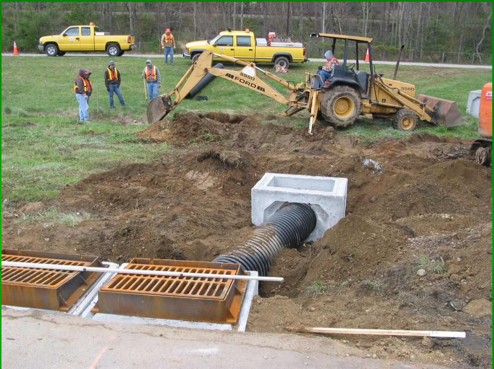
Excavating for Junction box below diversion box
