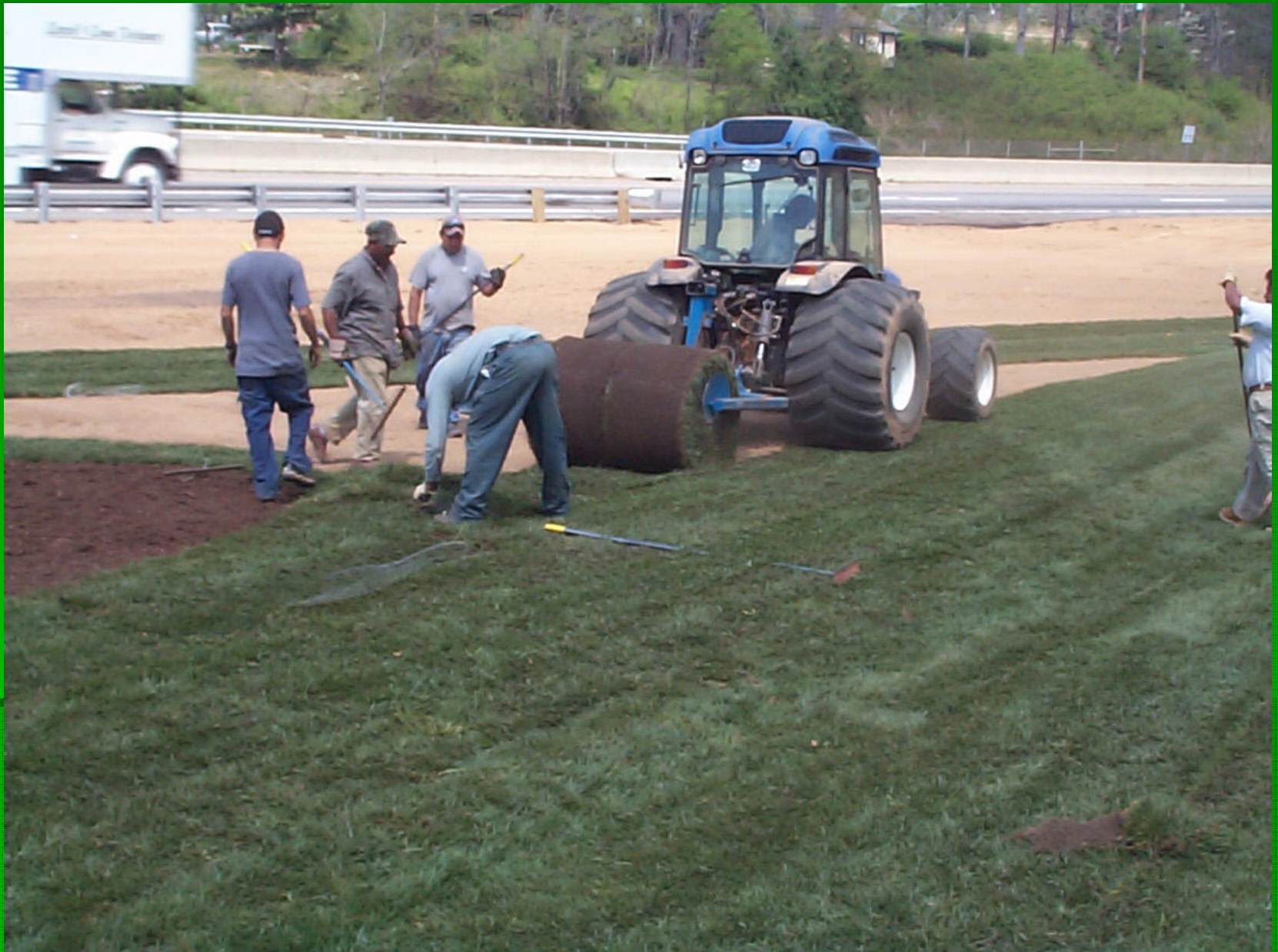
Sod Being Placed
