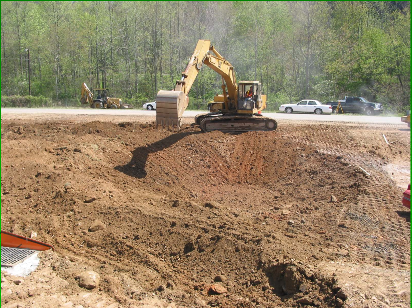
Excavation of Sediment Forebay
