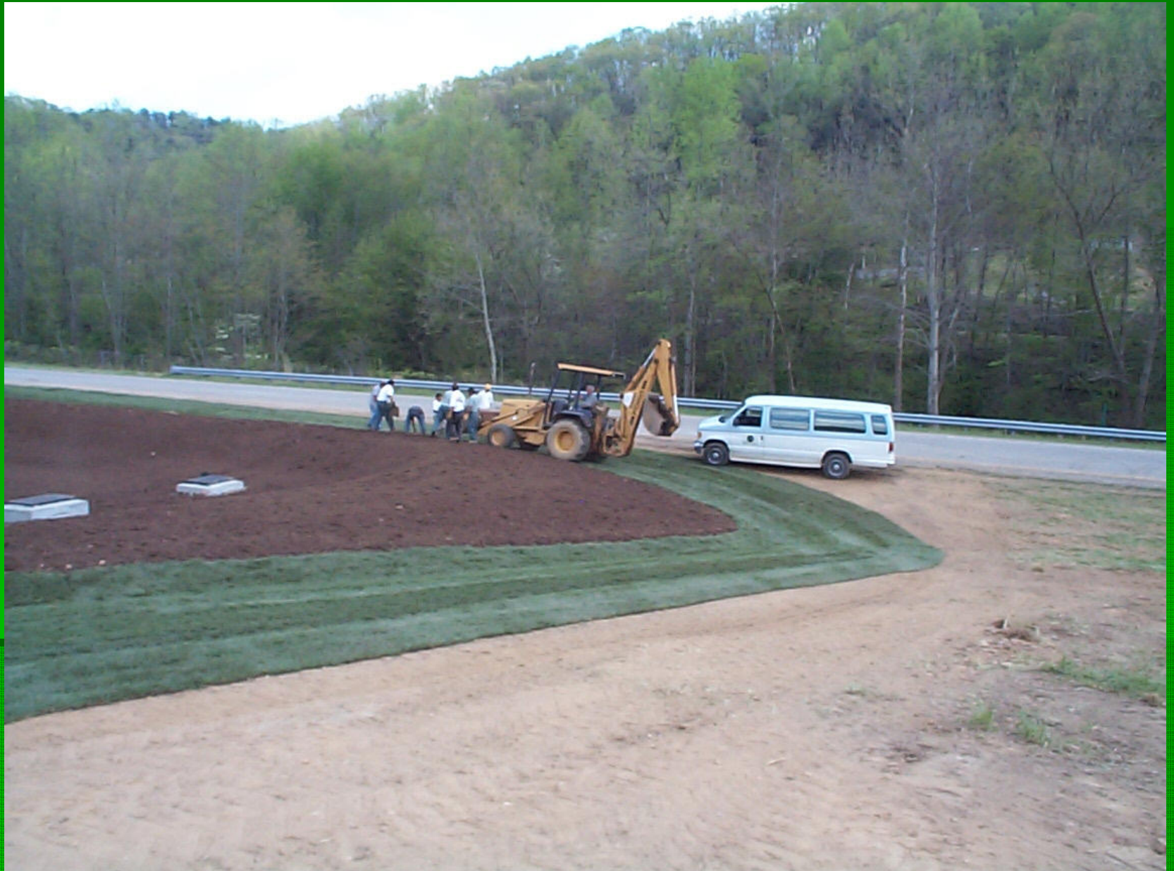
Lower edge of basin where berm ties to natural ground
