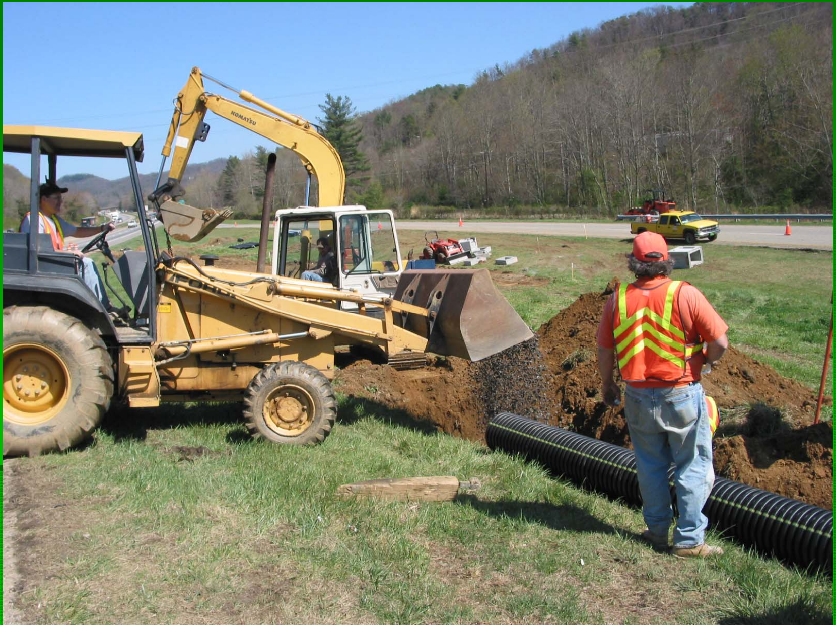
Pipe installation at Junction Box
