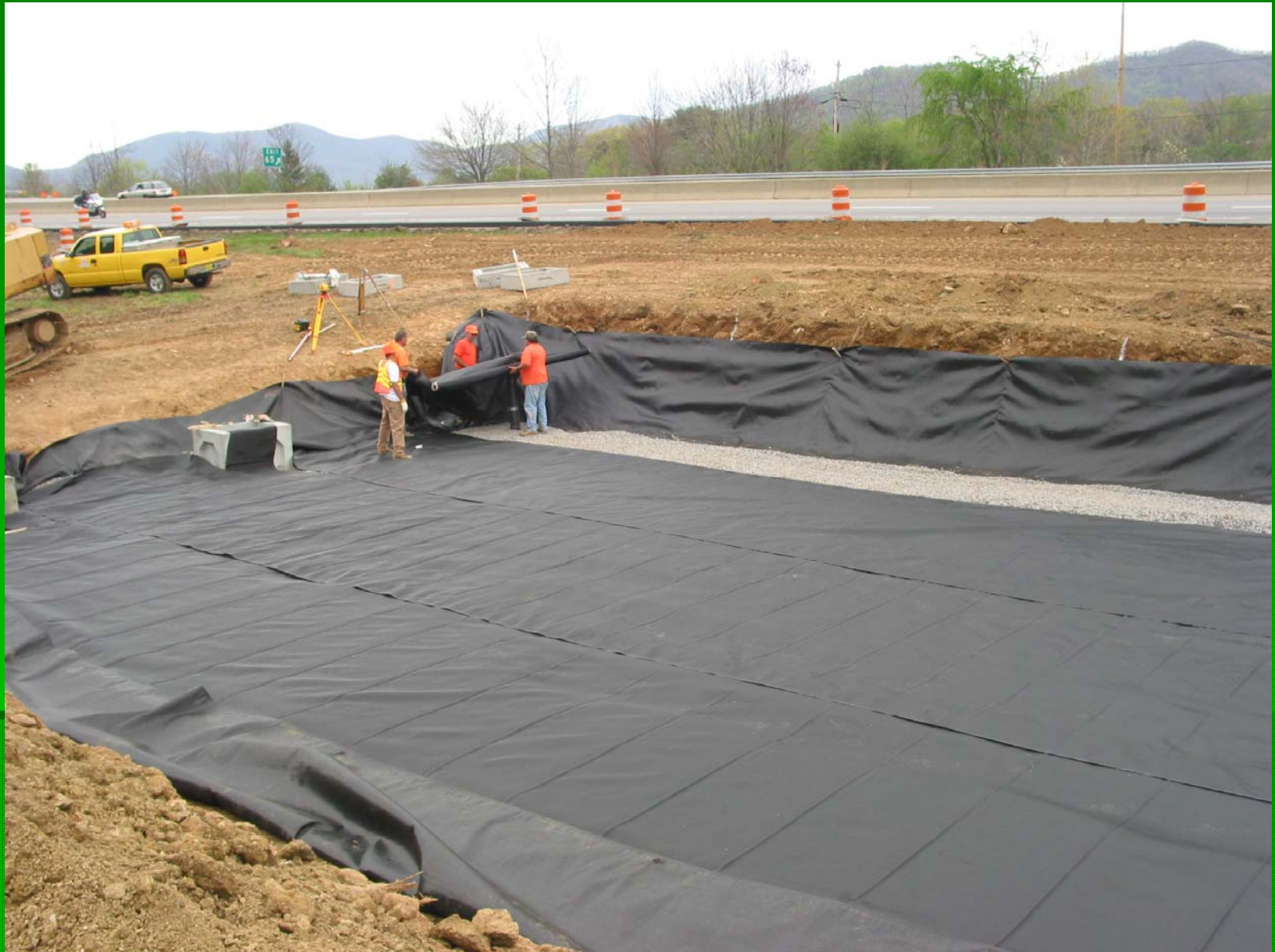
Geotextile Fabric Placed on Top of Stone
