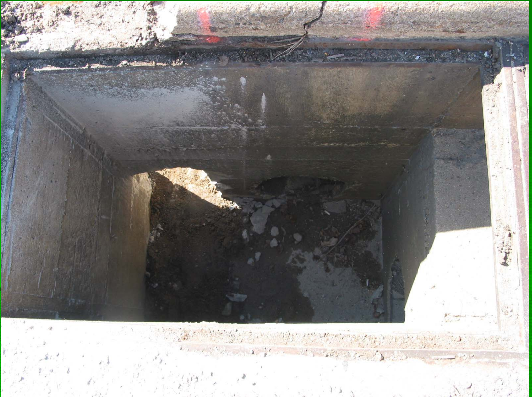
New outlet for diversion in upper drop inlet
