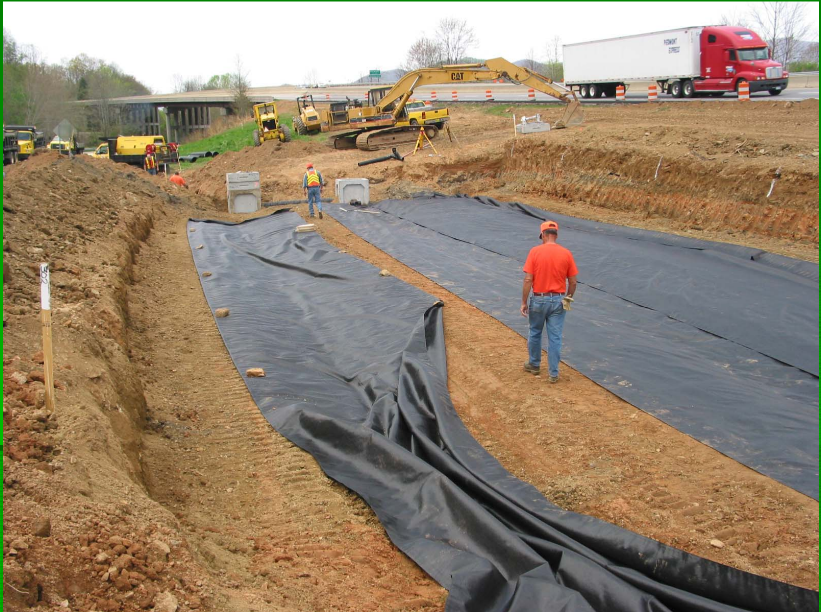
Geotextile Fabric Being Placed in Bottom of Basin
