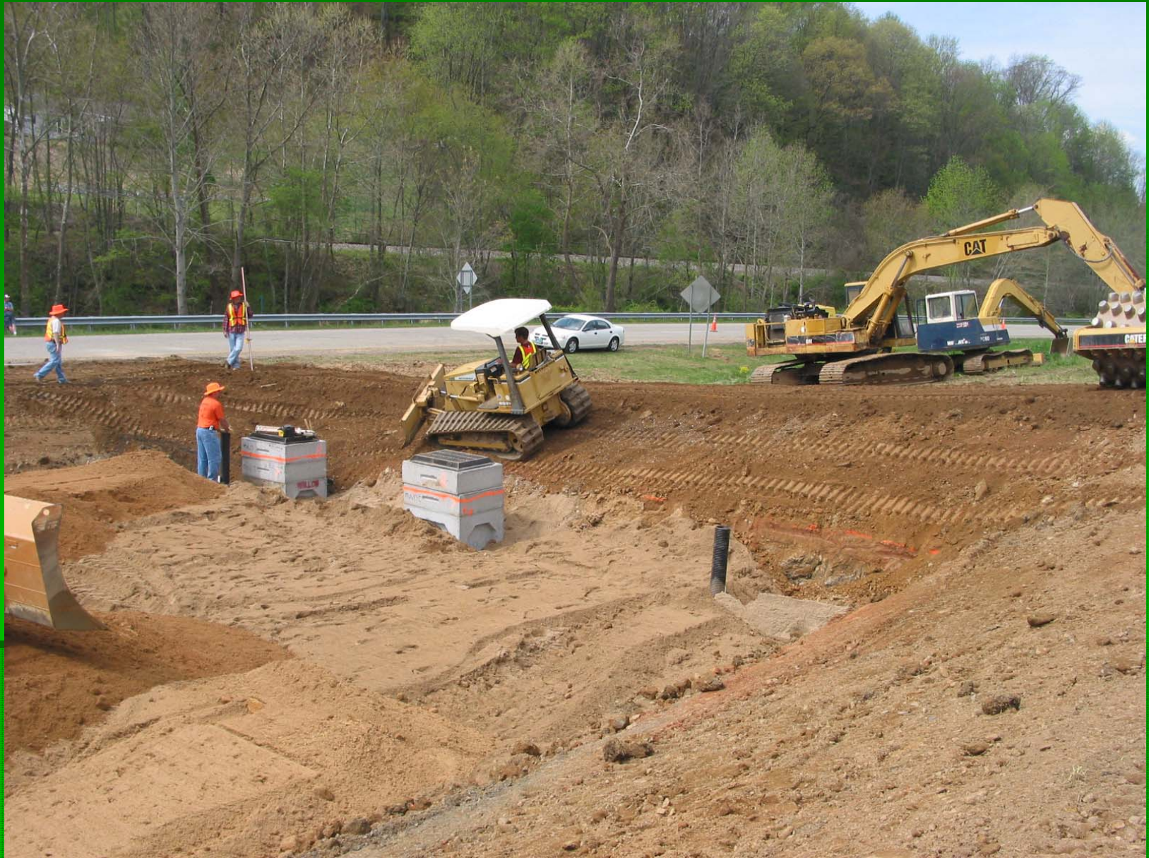
Finishing grade on side slopes
