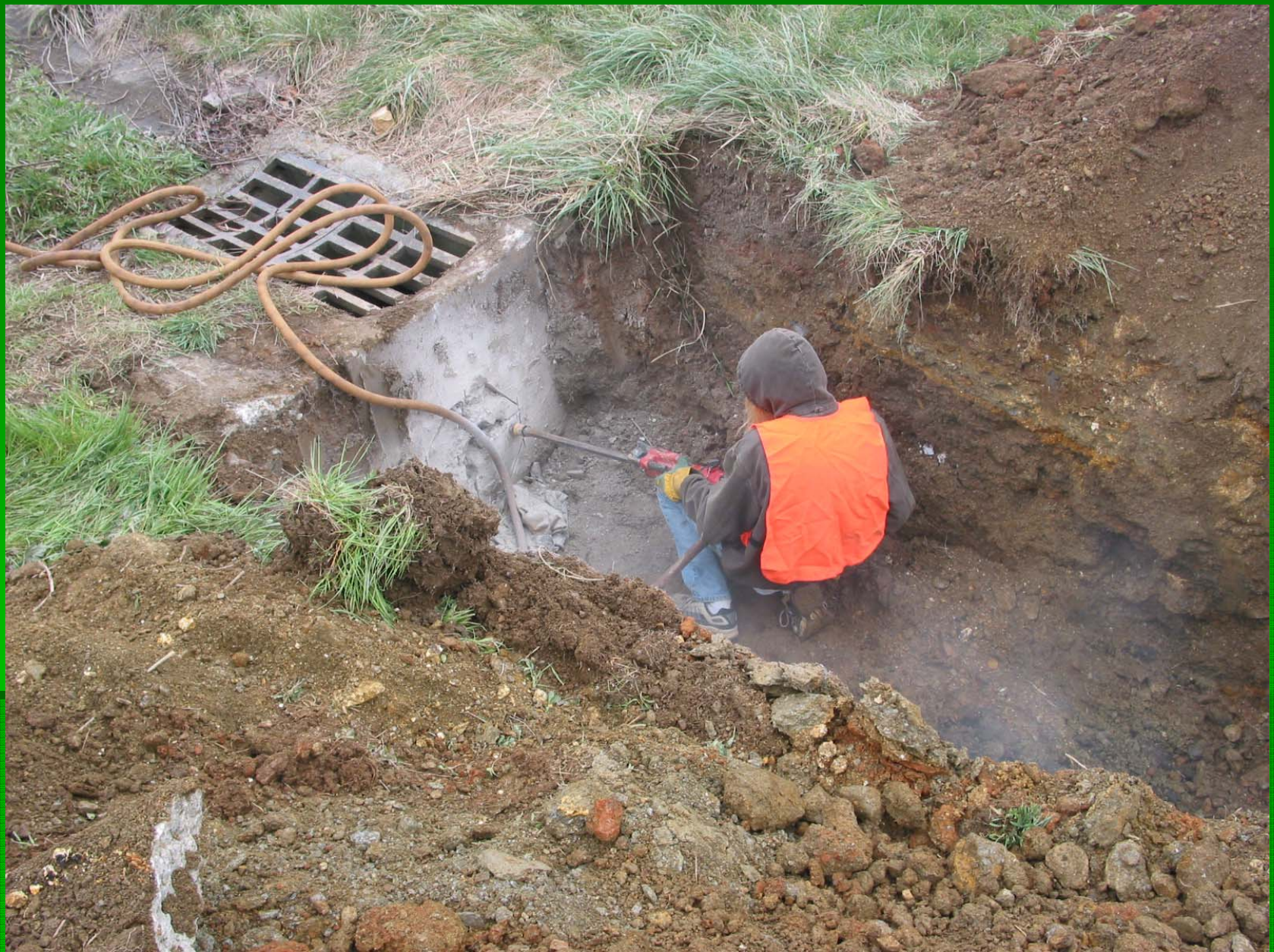
Drilling into existing Drop Inlet
