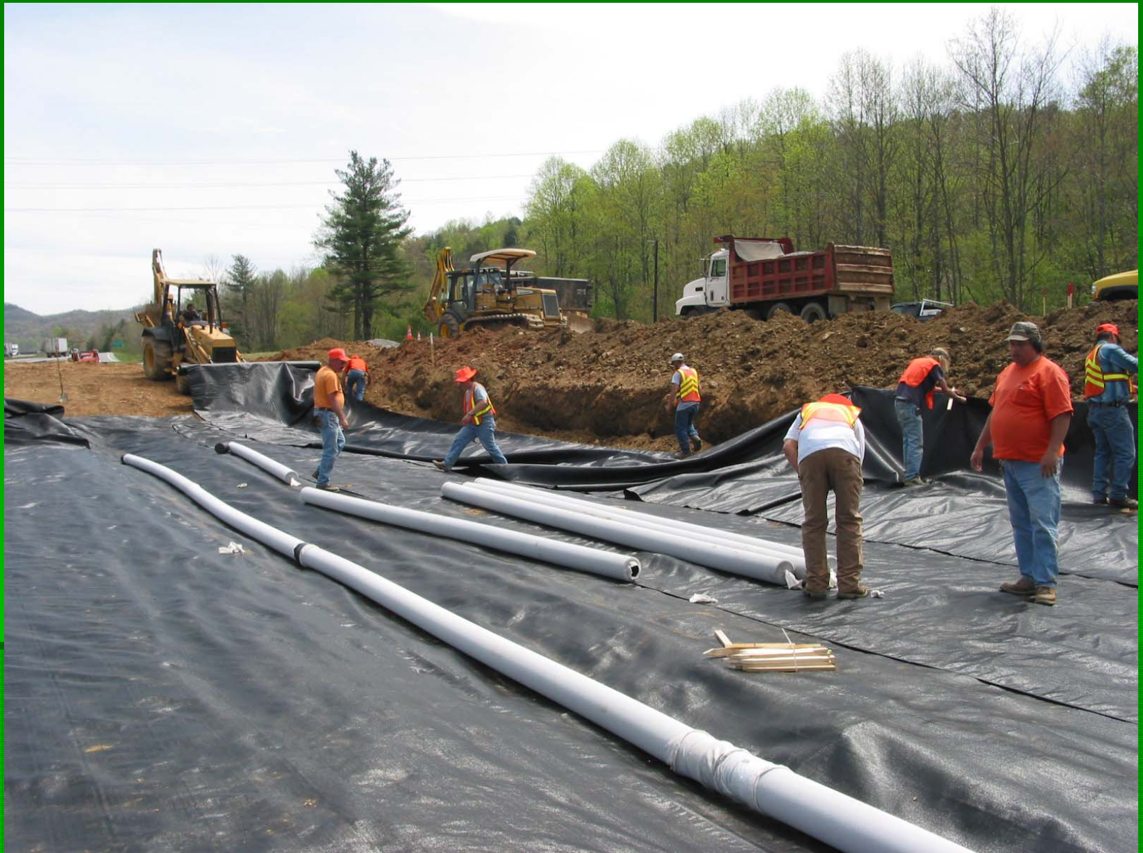
Underdrain perforated pipe being installed
