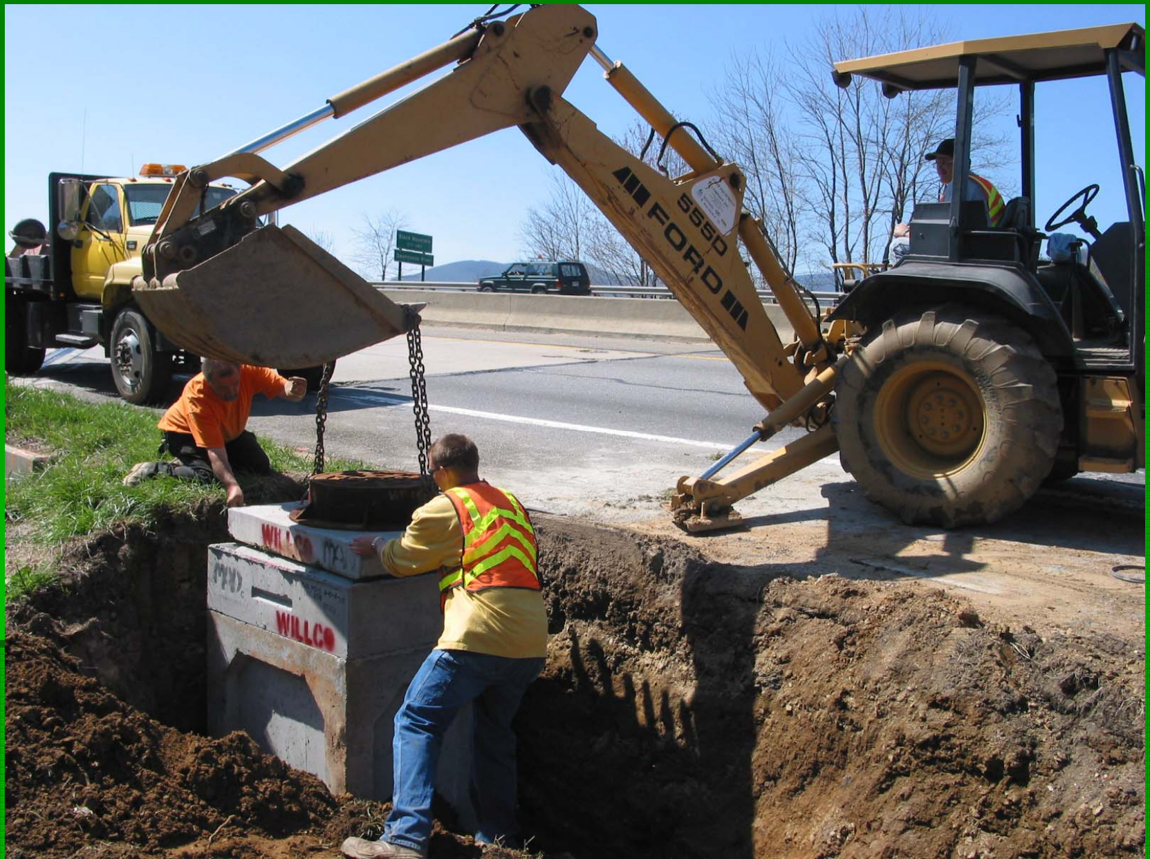
Installation of riser and manhole section on new junction box
