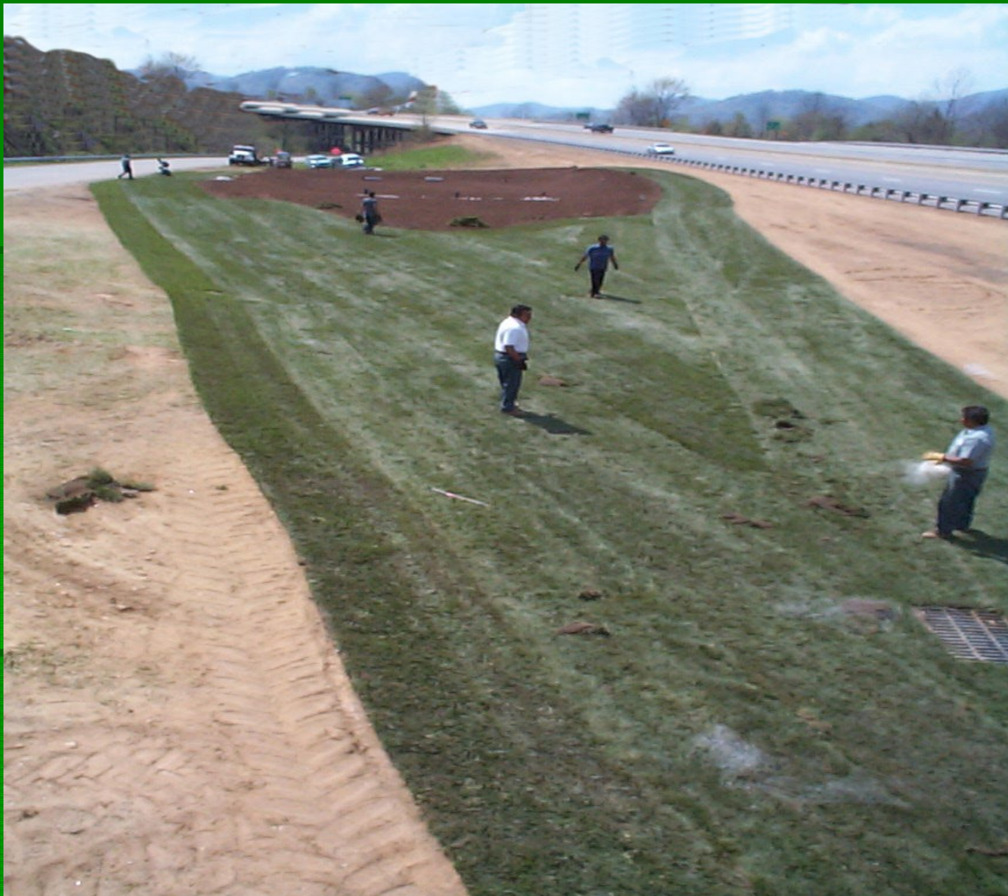
Finalizing sod around basin and drop inlet
