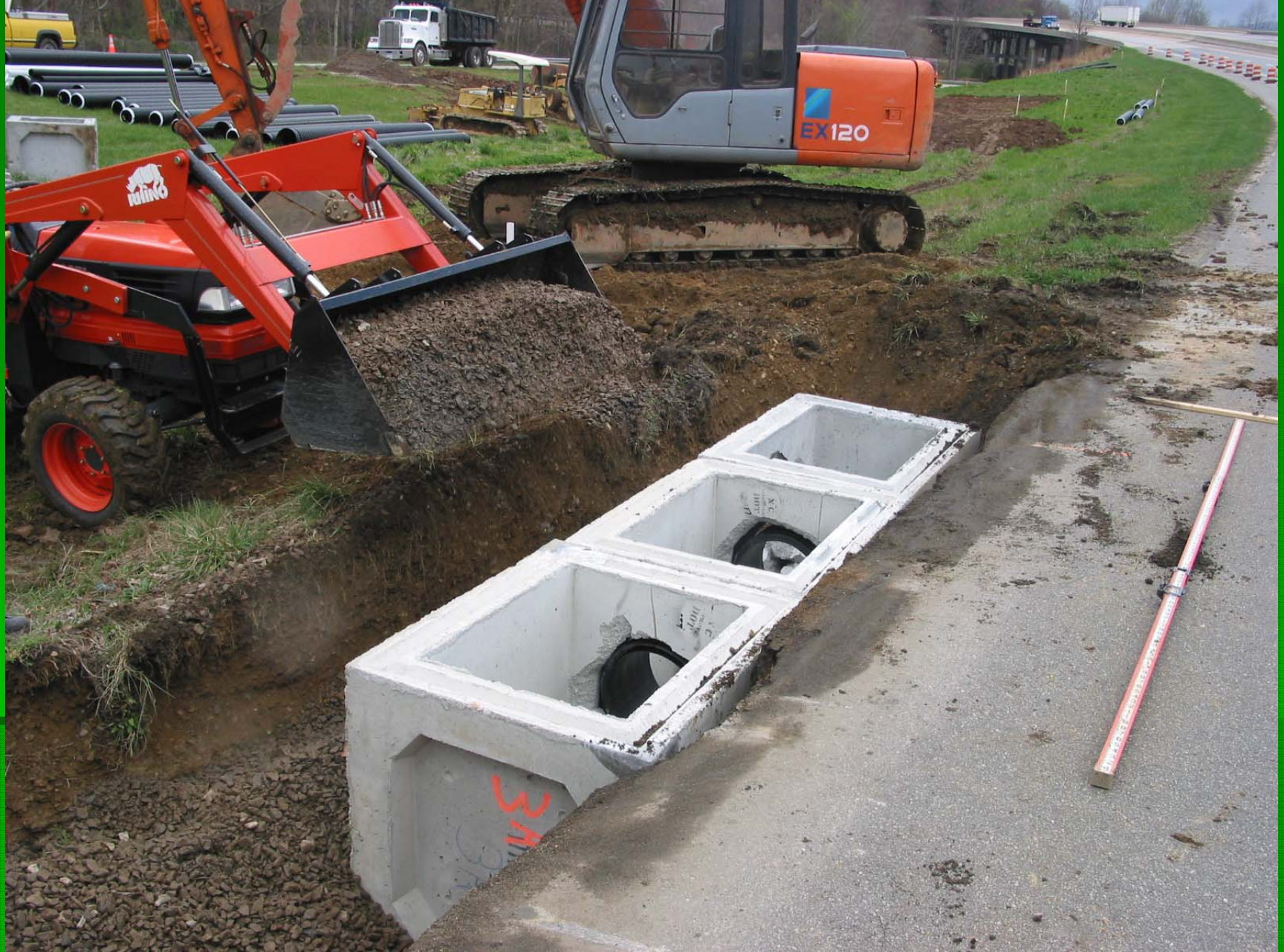
Catch basins in place, backfill with #57 stone.
