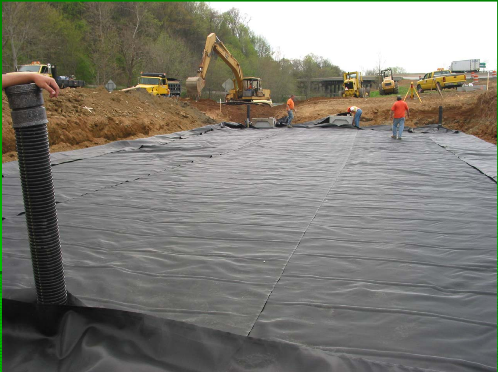
Finish grade for Engineered back fill material
