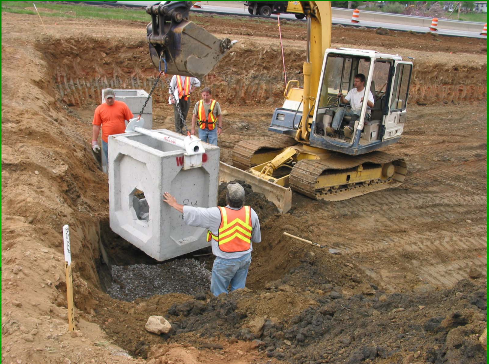
Installation of interior drop inlet inside basin
