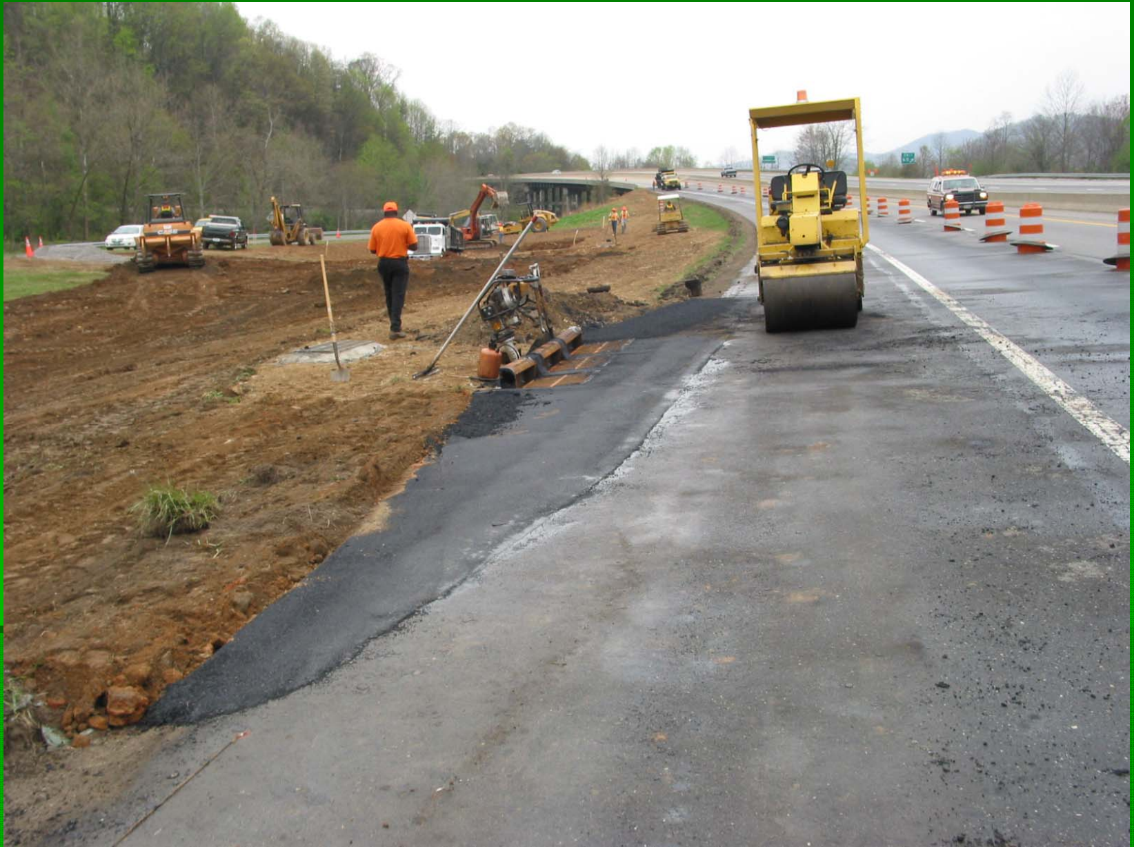
Compacting Asphalt
