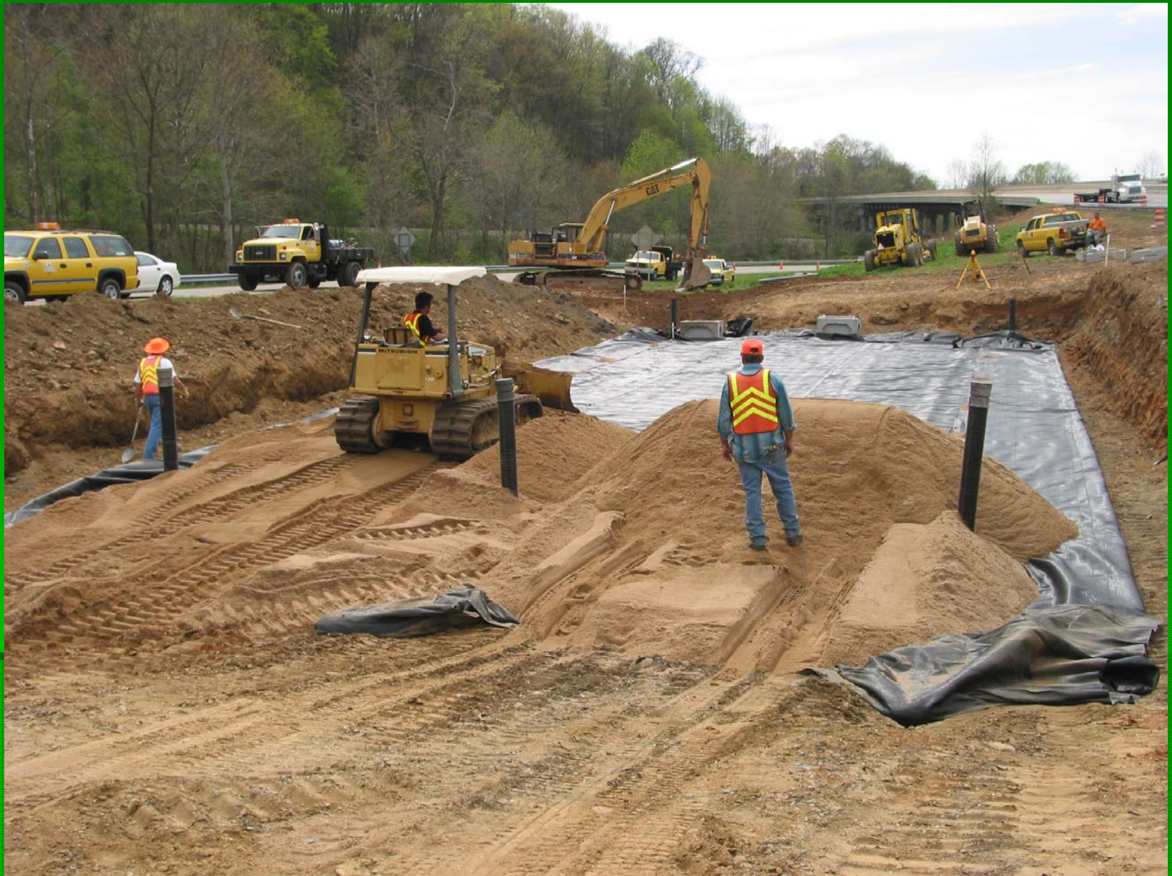
Placing engineered soil in lifts
