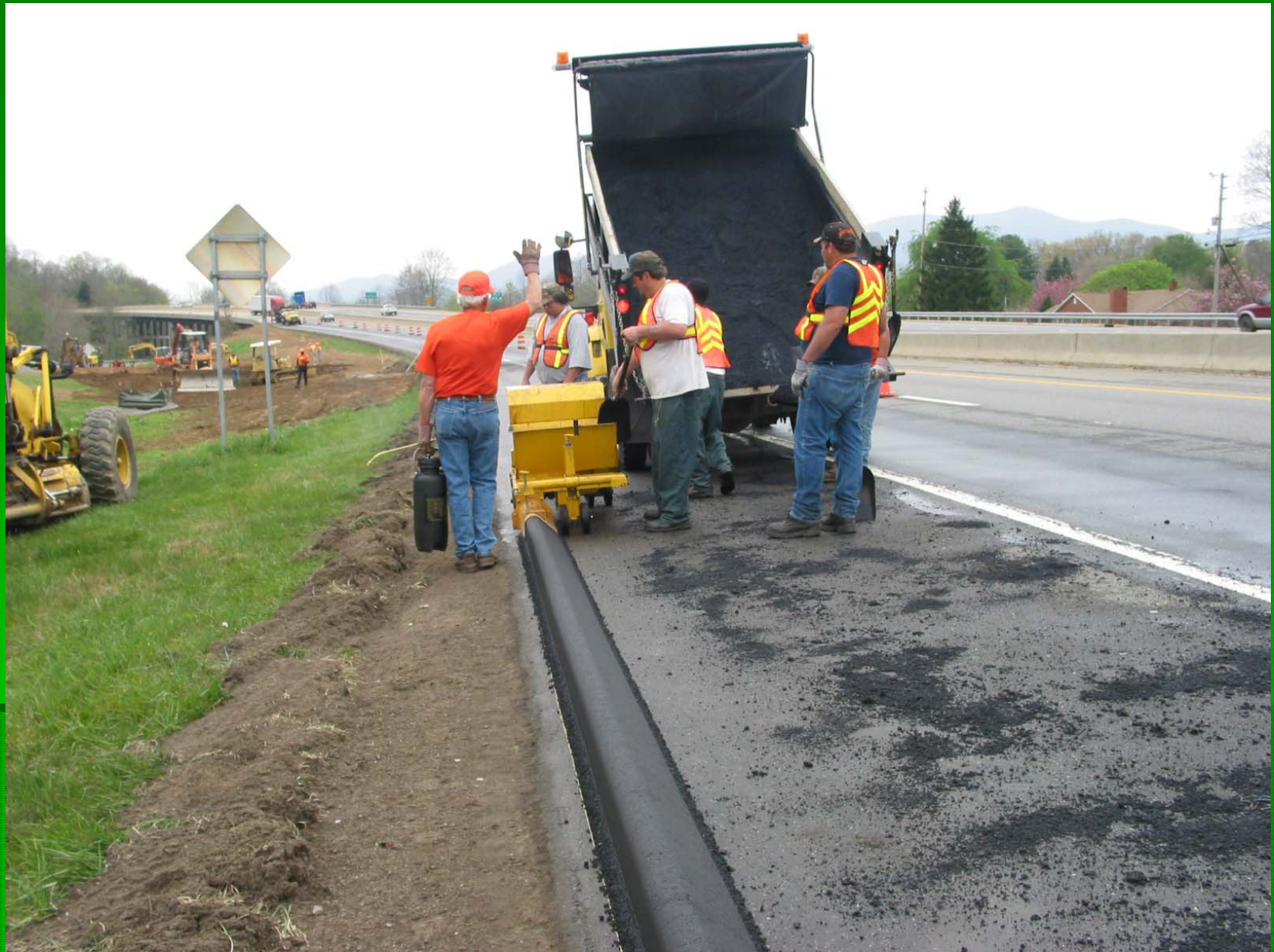
Asphalt Curb Being Formed
