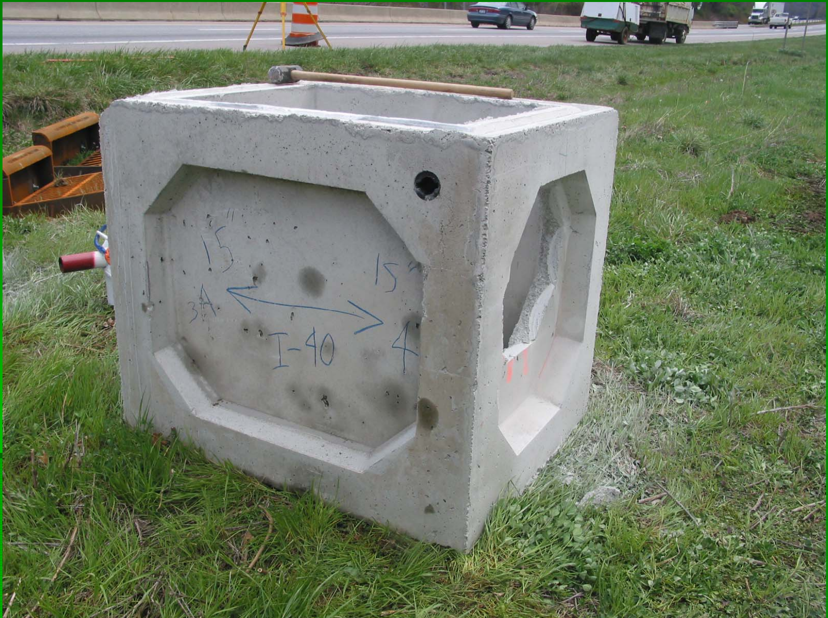
Precast catch basin to be installed along I-40 East
