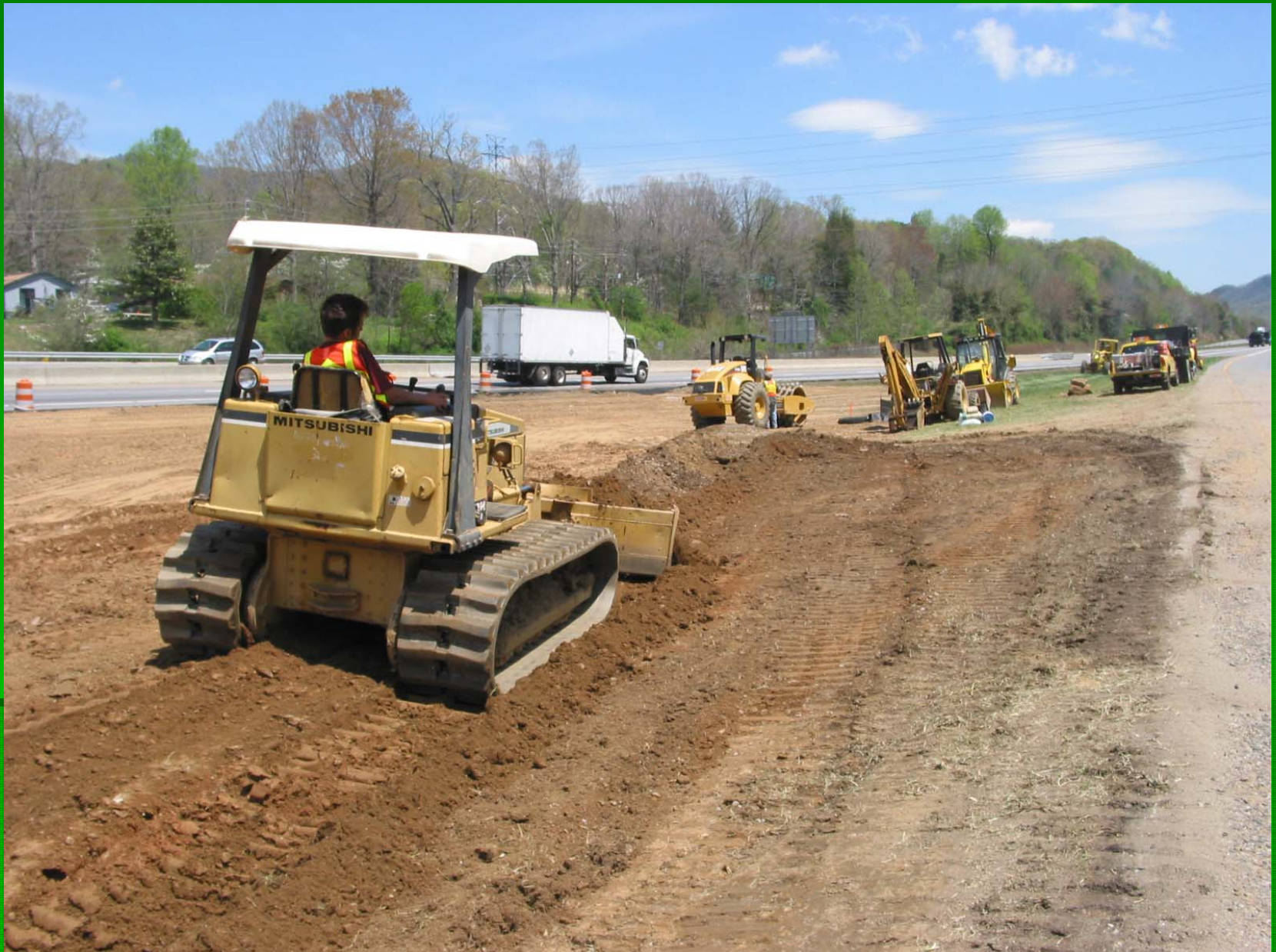
Constructing diversion berm around perimeter of basin
