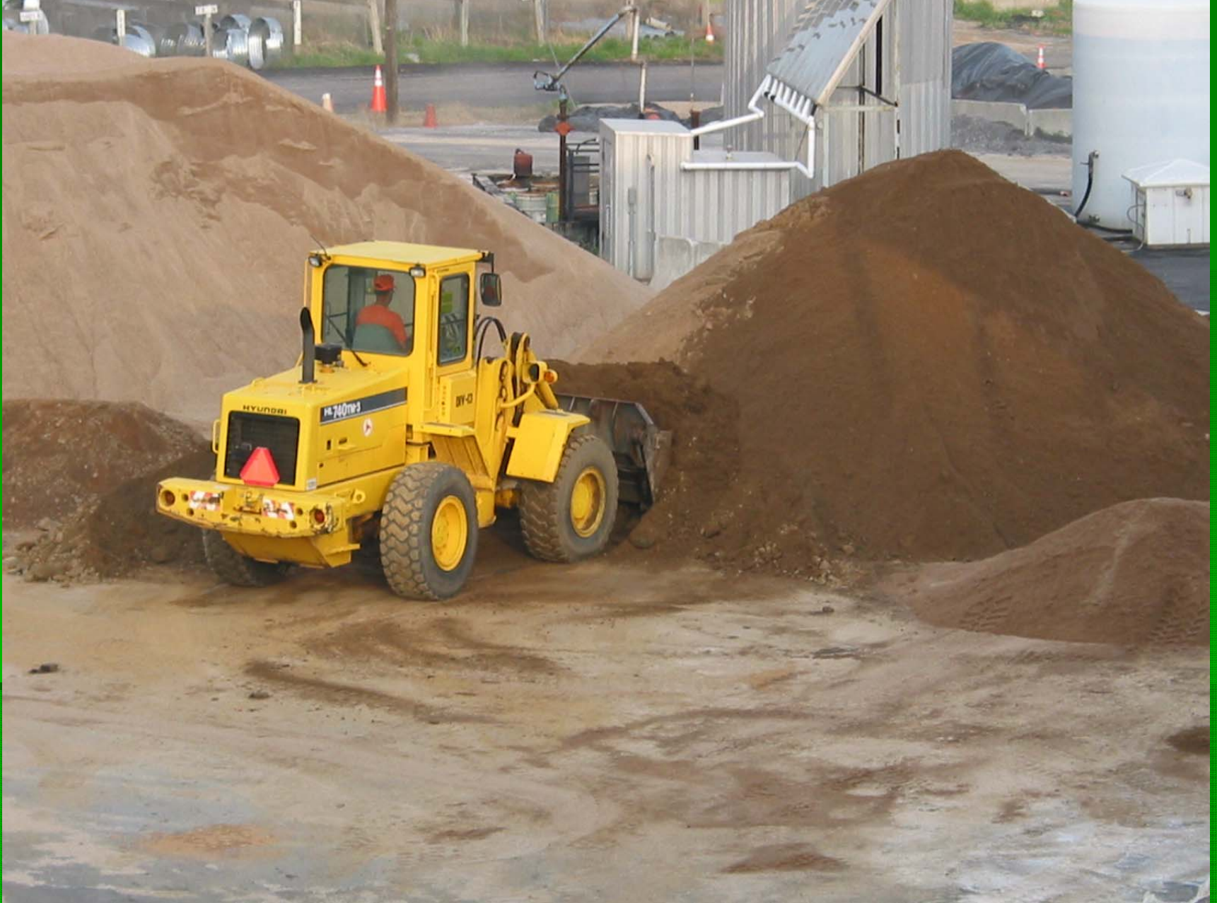
Mixing of Engineered Soil, 70% - 30% Ratio
