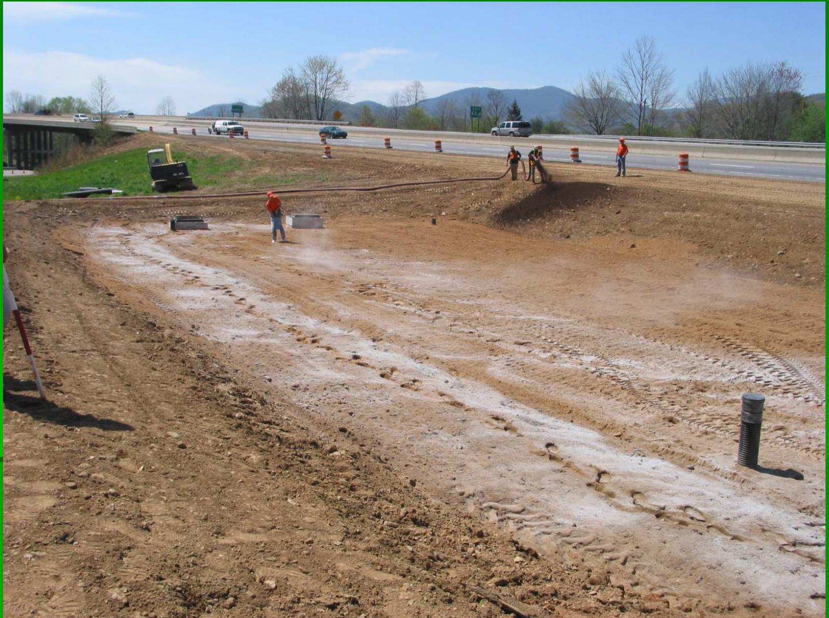
Lime and Nutrients Spread Prior to Mulching and Planting
