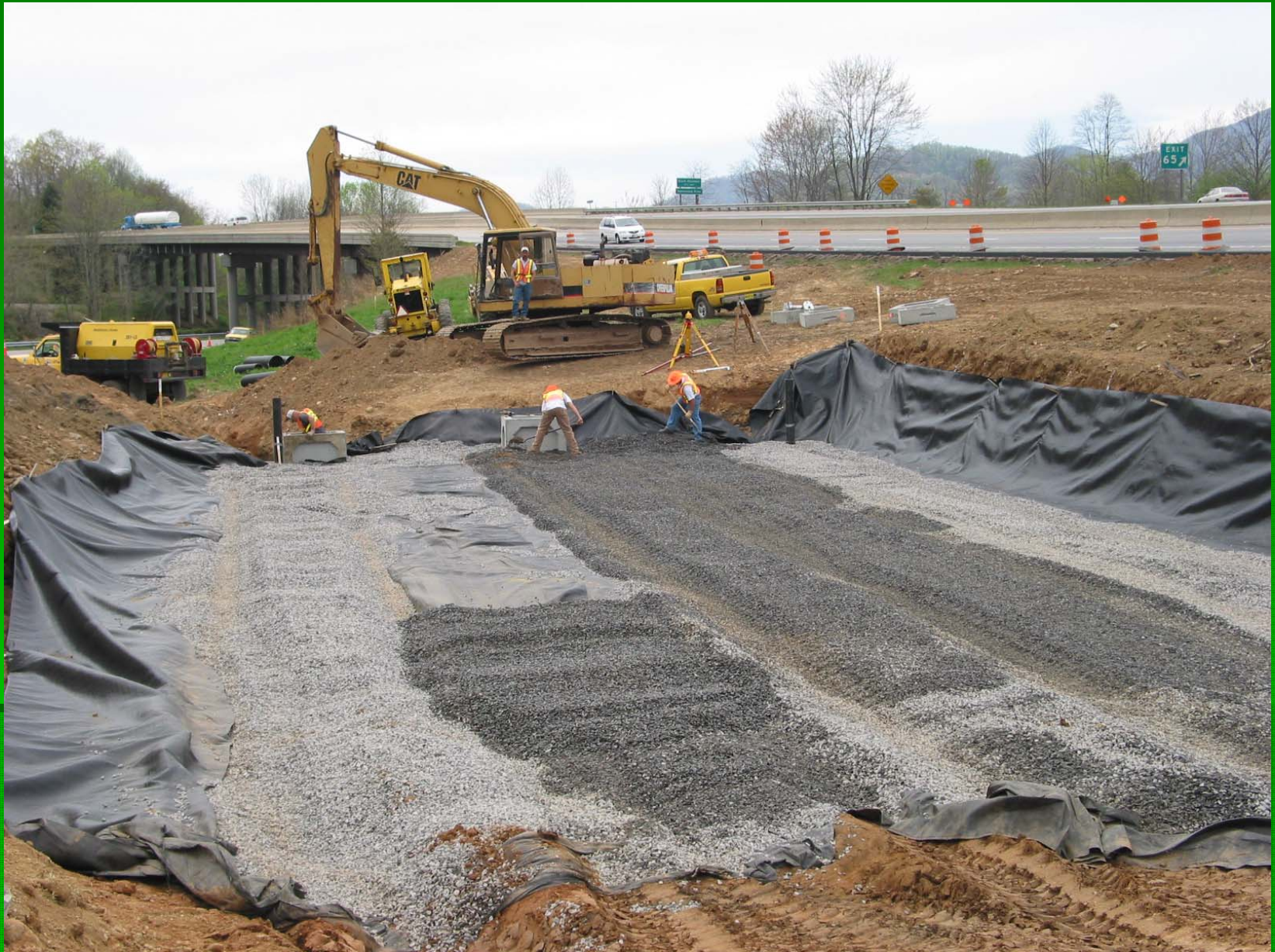
Placing Stone in Basin over underdrain pipe
