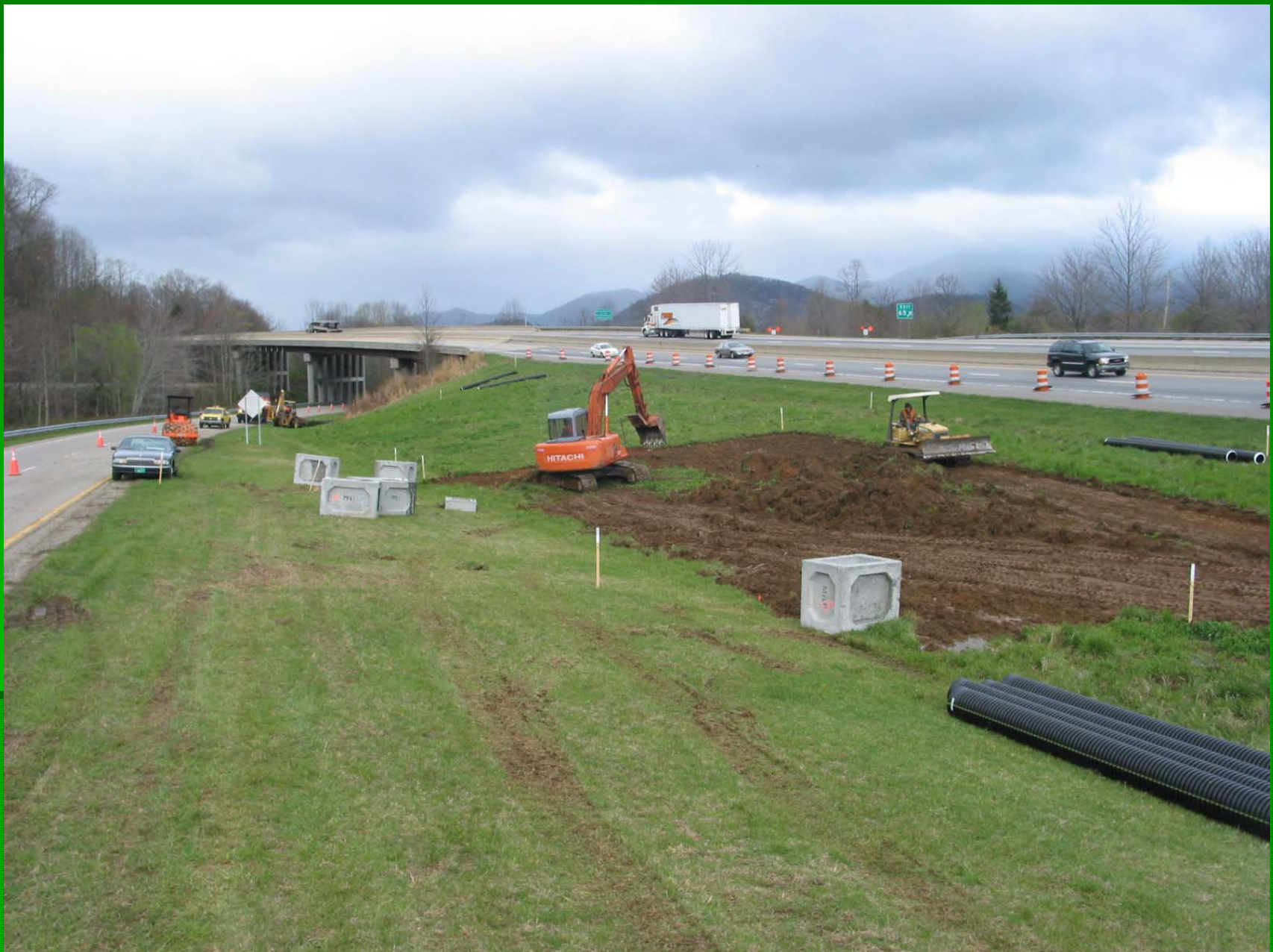
Removing Top soil in Basin Area
