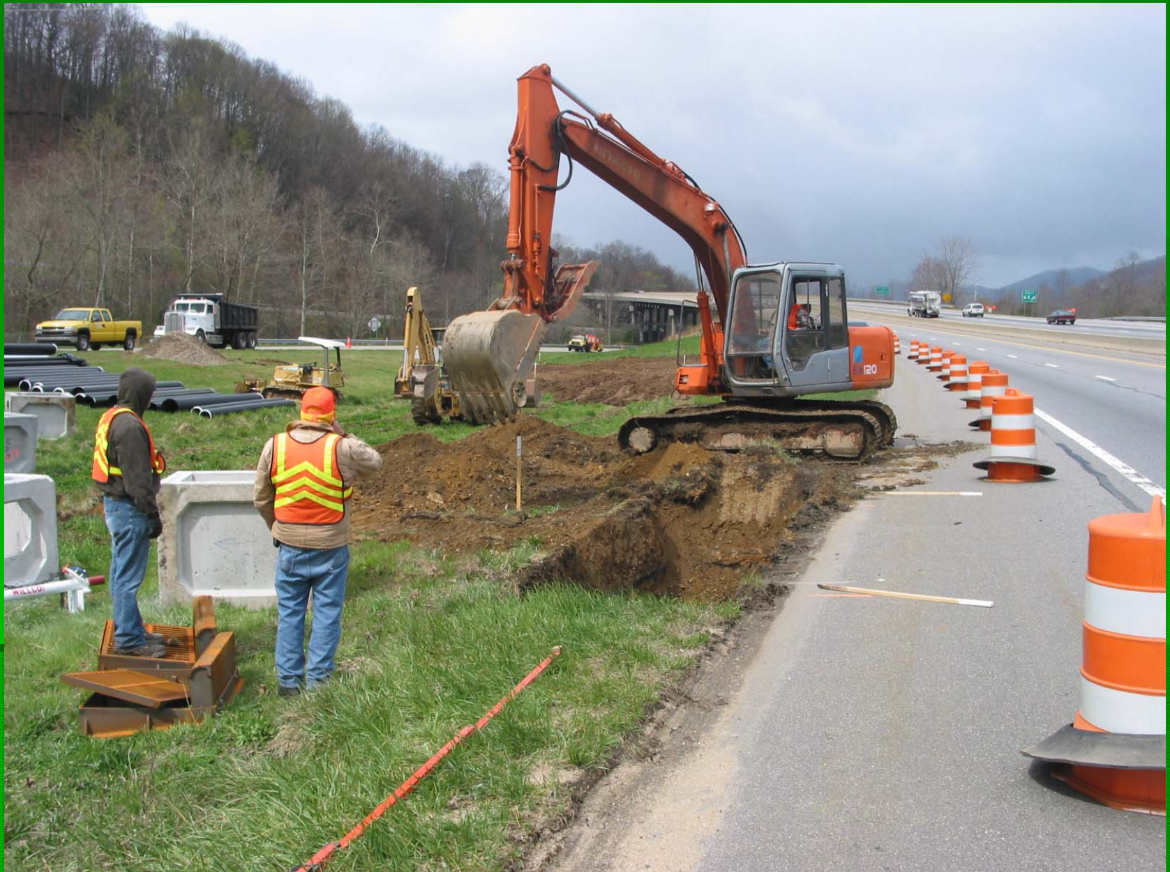
Excavating for the 3 catch basin to be installed along the curb line.
