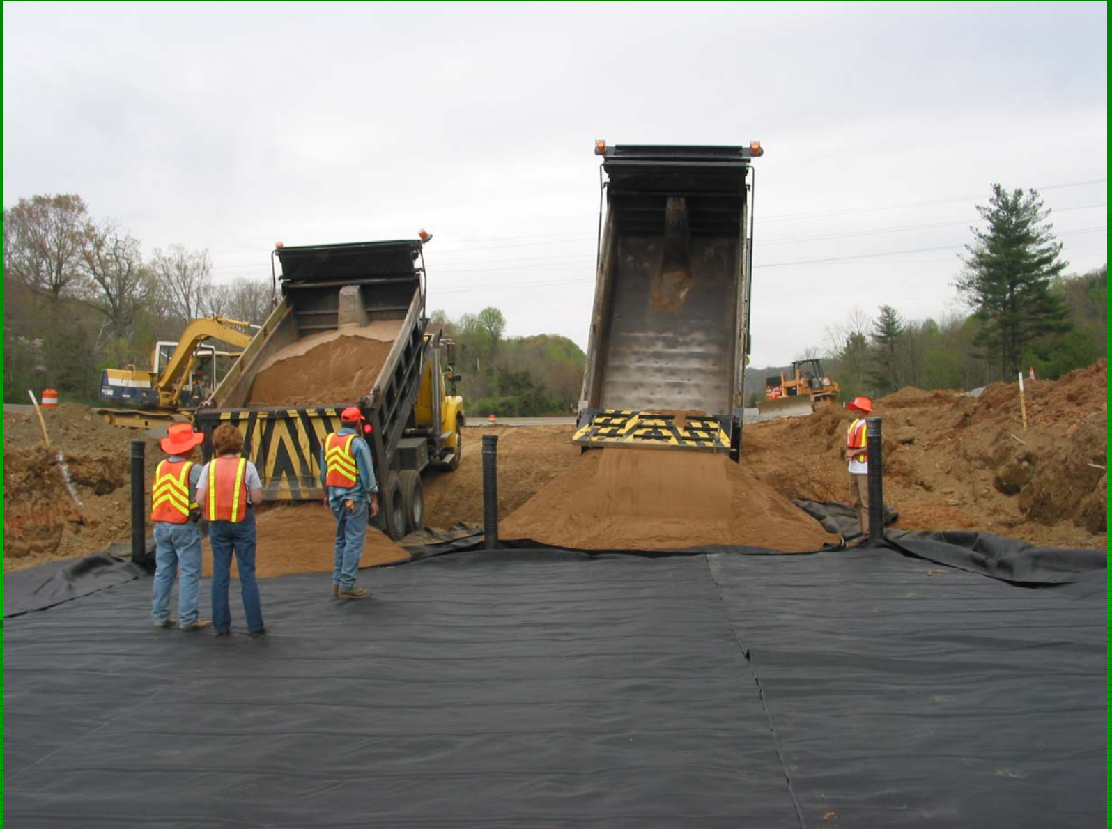
Placing of Engineered Soil / Sand
