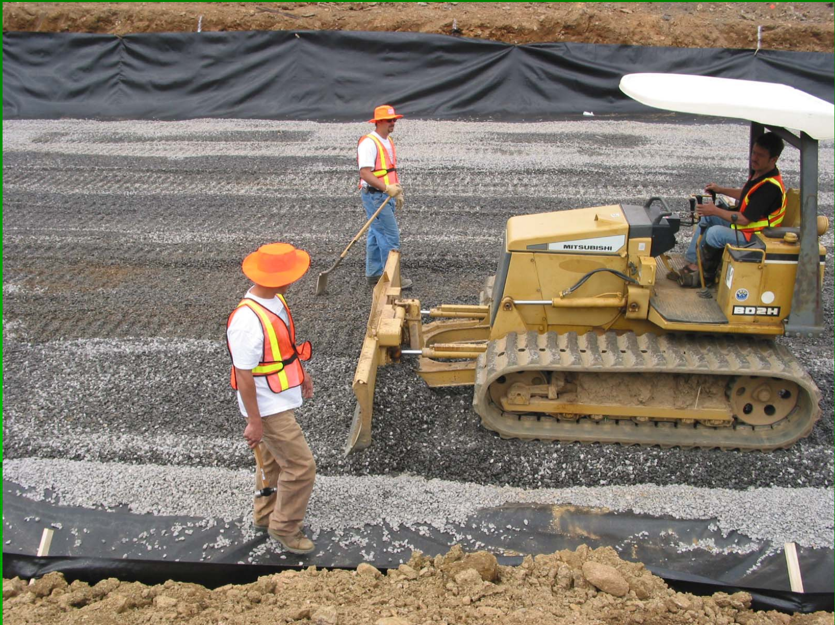
Finish grade of stone over underdrain pipe
