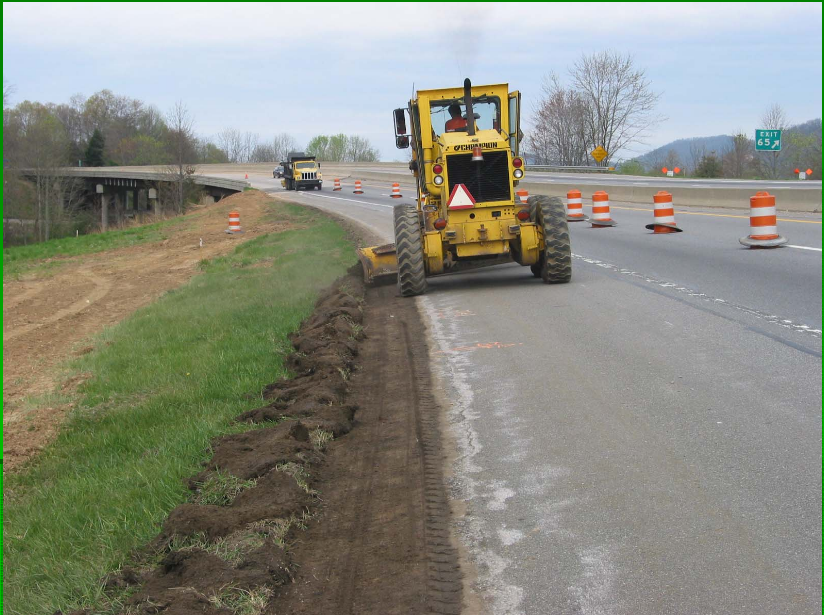
Shoulder Being Prepared for Curb
