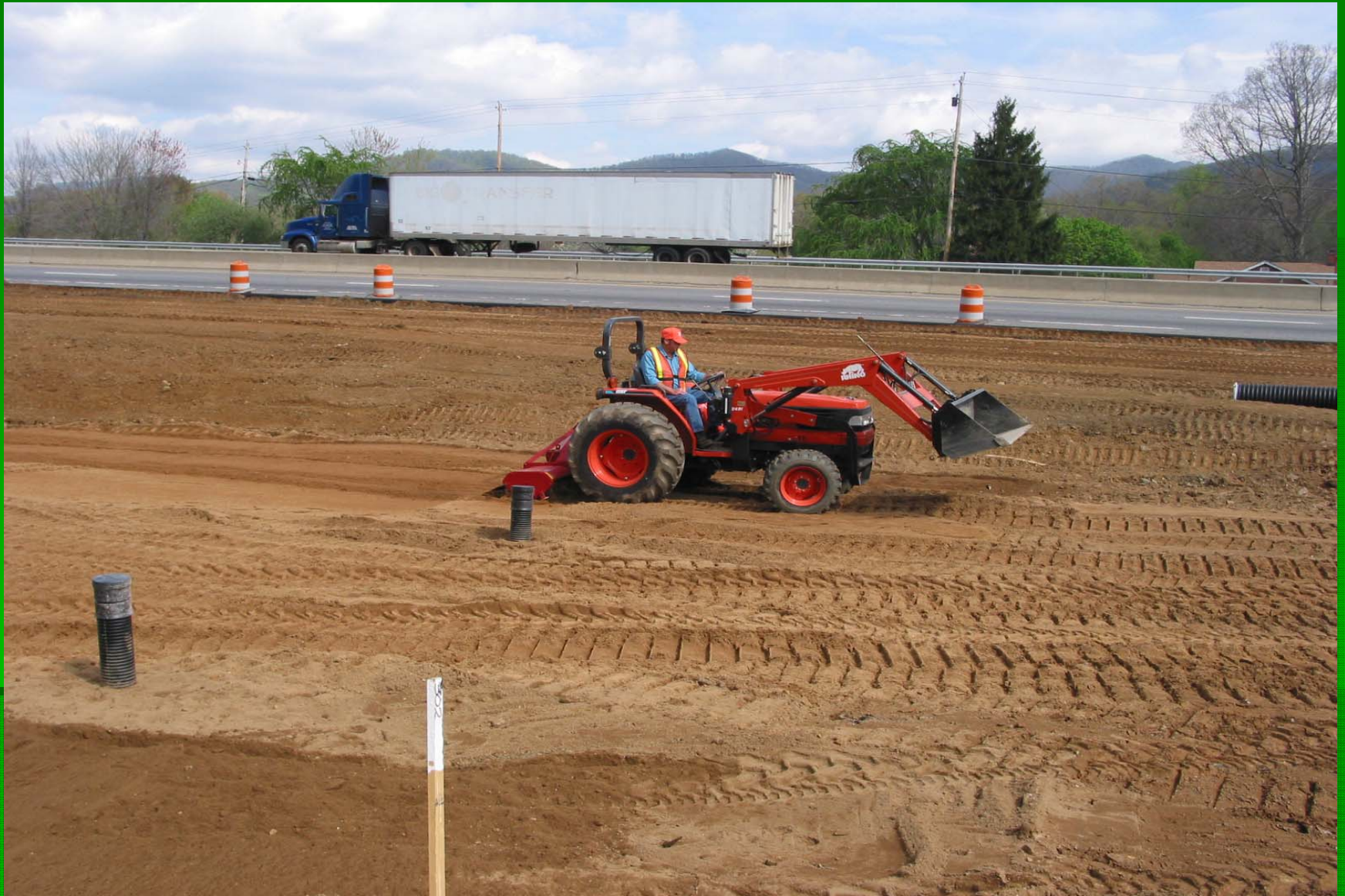
Roto tilling mix for consistency in material
