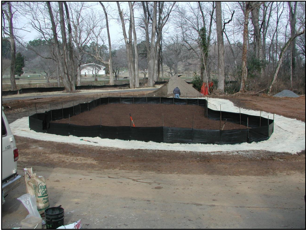
Figure 8.1. Silt Fence Around the Perimeter to Protect From Sedimentation
