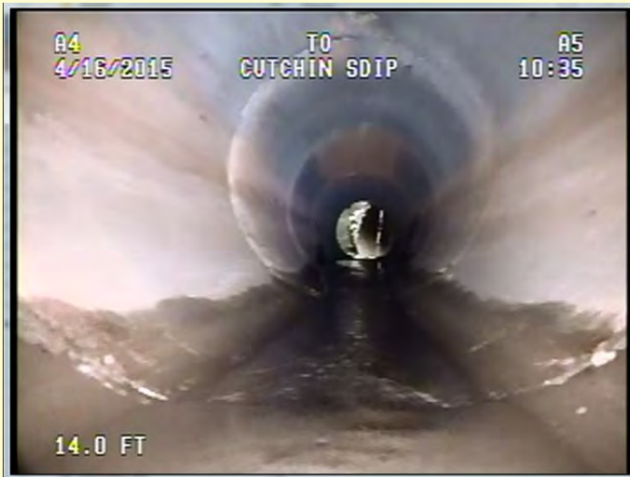
Example of a pipe in good condition
