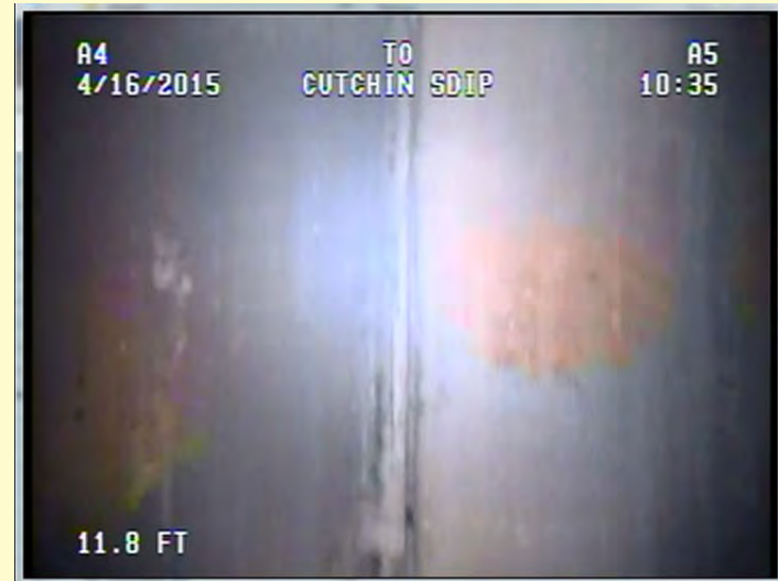
Example of a pipe joint in good condition
