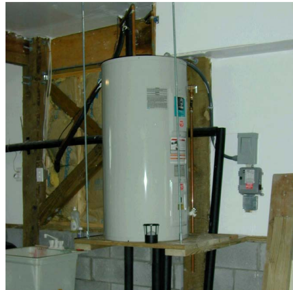
Figure 31: Example of Elevated Utilities
