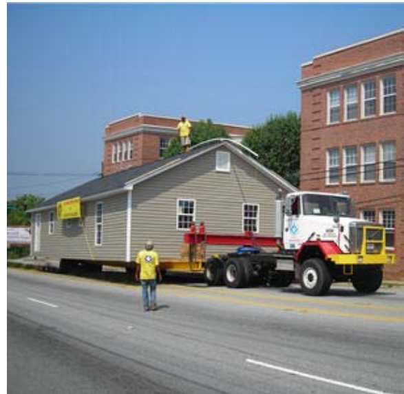
Figure 18: Example of House Relocation
