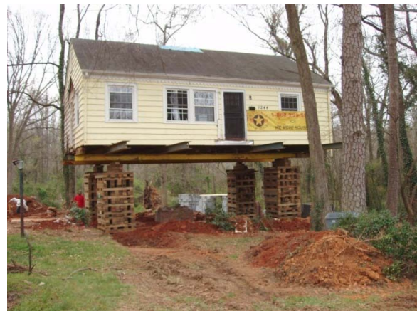
Figure 19: House During Elevation Process
