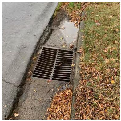
Existing catch basin along Grier Road with ponding occurring STA 12+50
