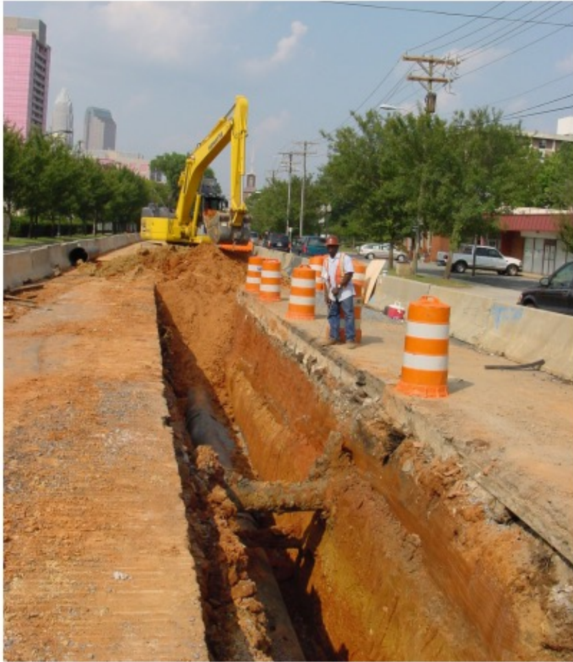
24-inch drinking water pipe installation.
