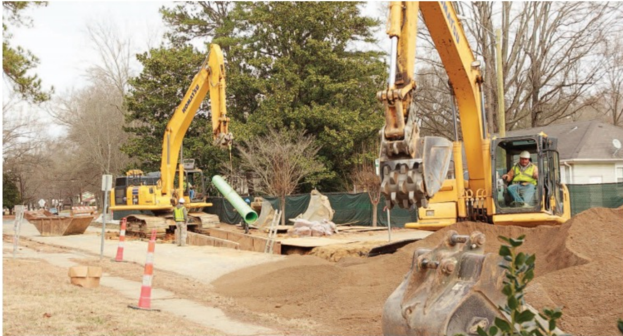
24-inch wastewater pipe project under a street.
