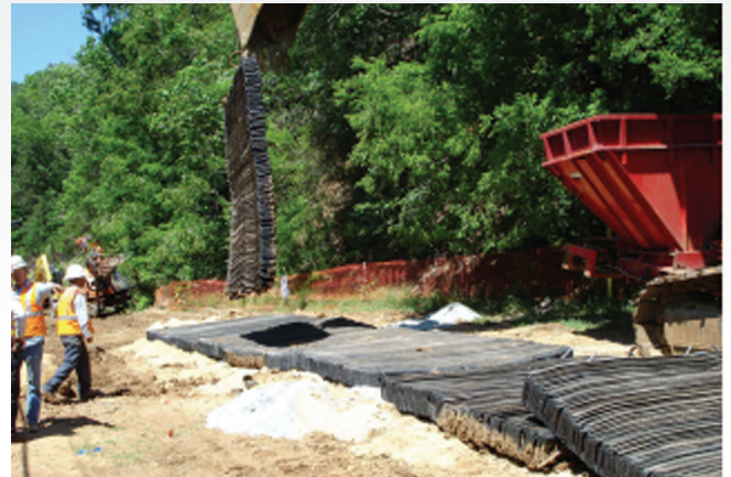
Heavy mats are placed on the blasting area to control impact.
