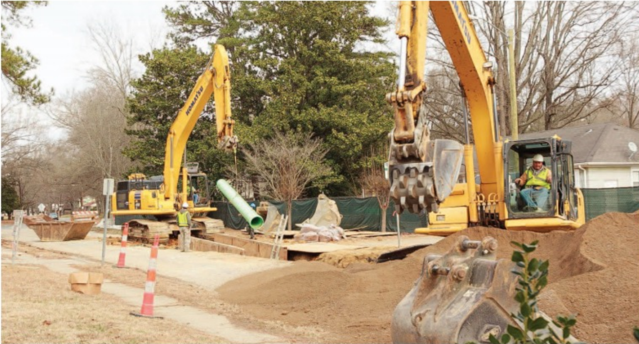
24-inch wastewater pipe project under a street.
