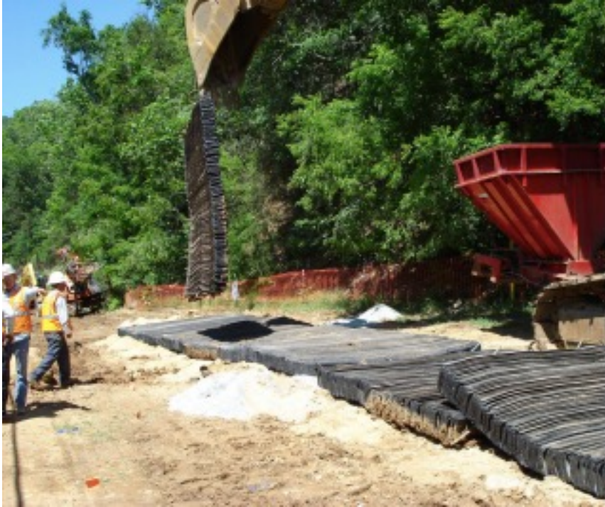
Heavy mats are placed on the blasting area to control impact.
