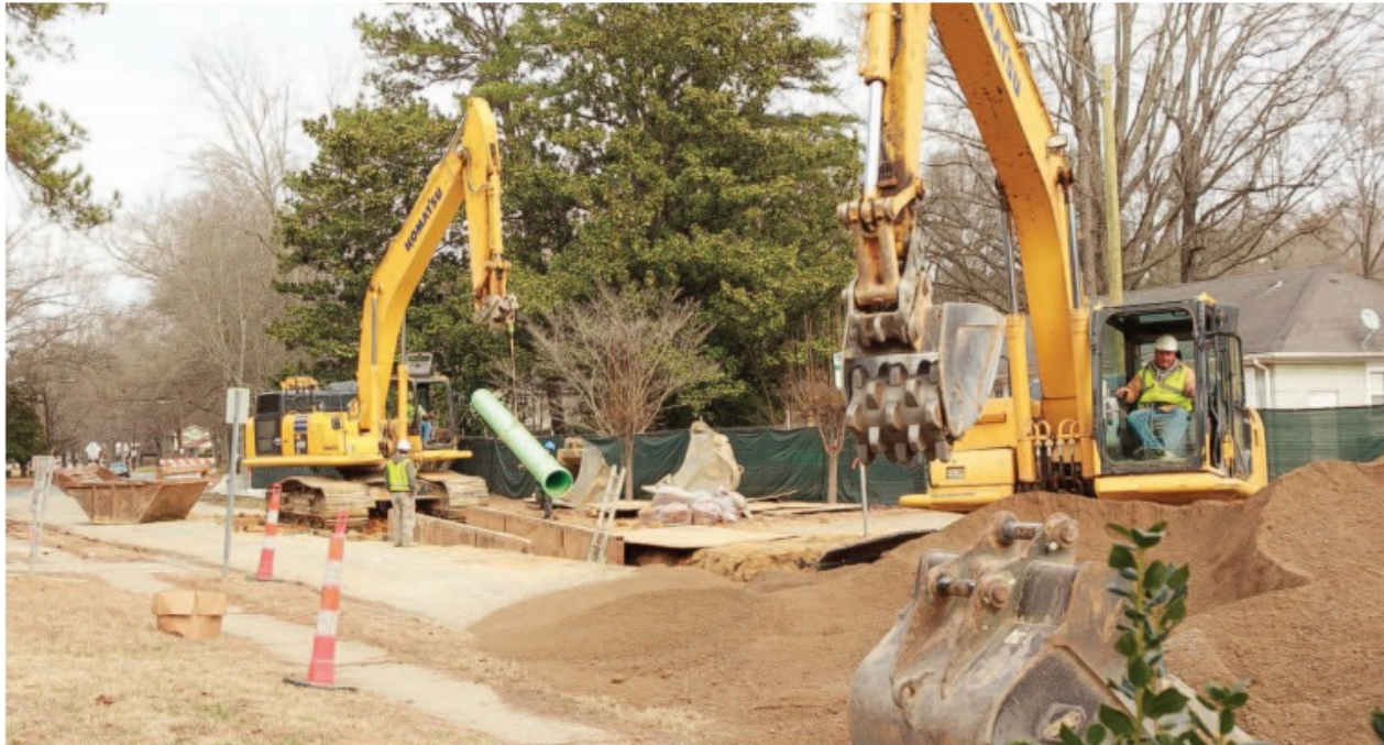
24-inch wastewater pipe project under a street.
