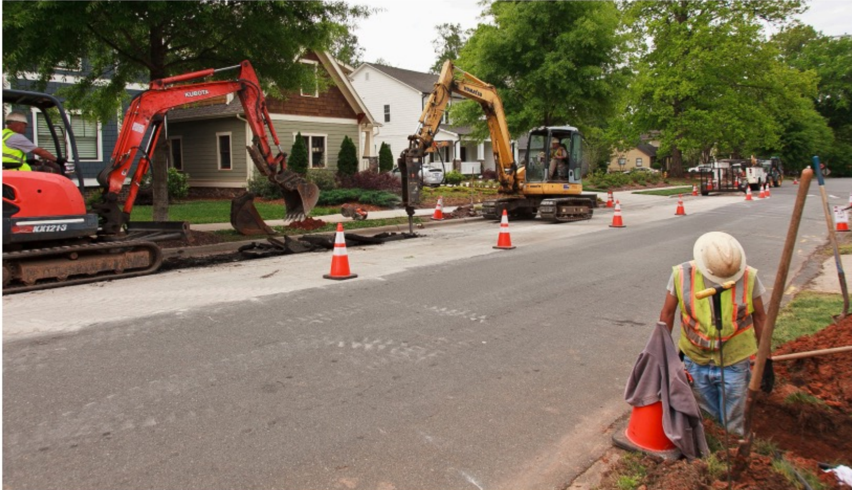
6-inch drinking water pipe replacement project including new service pipes to each water meter.
