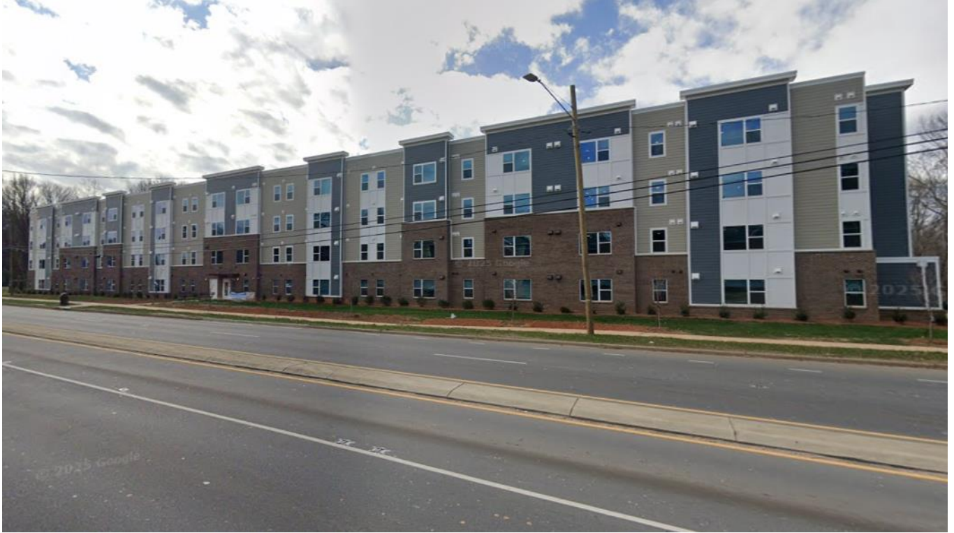
View of a new multi-family development located at the southwest corner of East WT Harris Boulevard and Wallace Avenue, southwest of the site.
