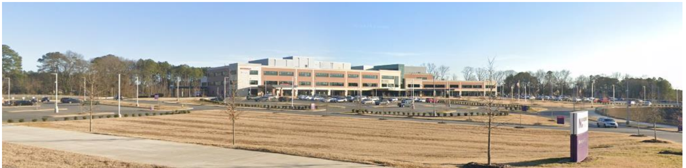
Street view of the site as seen from Providence Road West.
