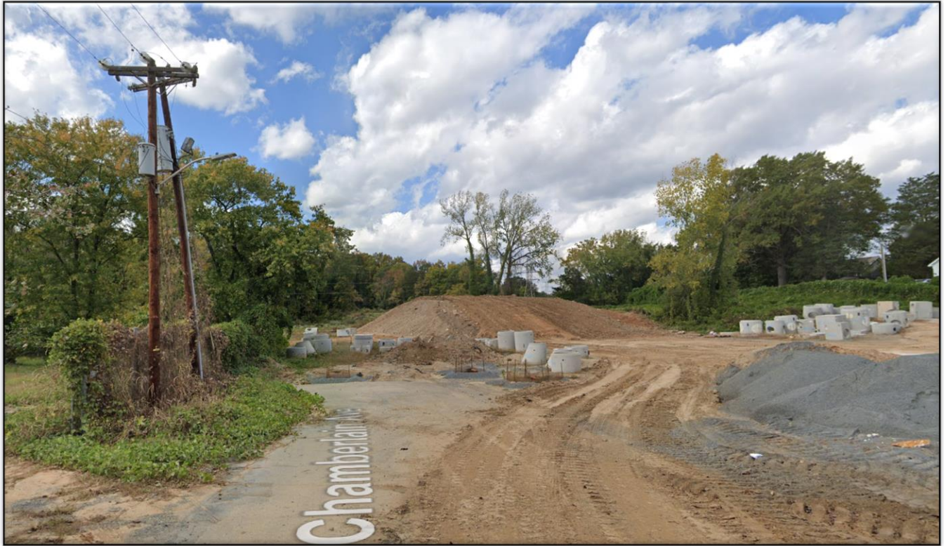
Located to the north of the site is a vacant lot with a greenway and park beyond the lot.
