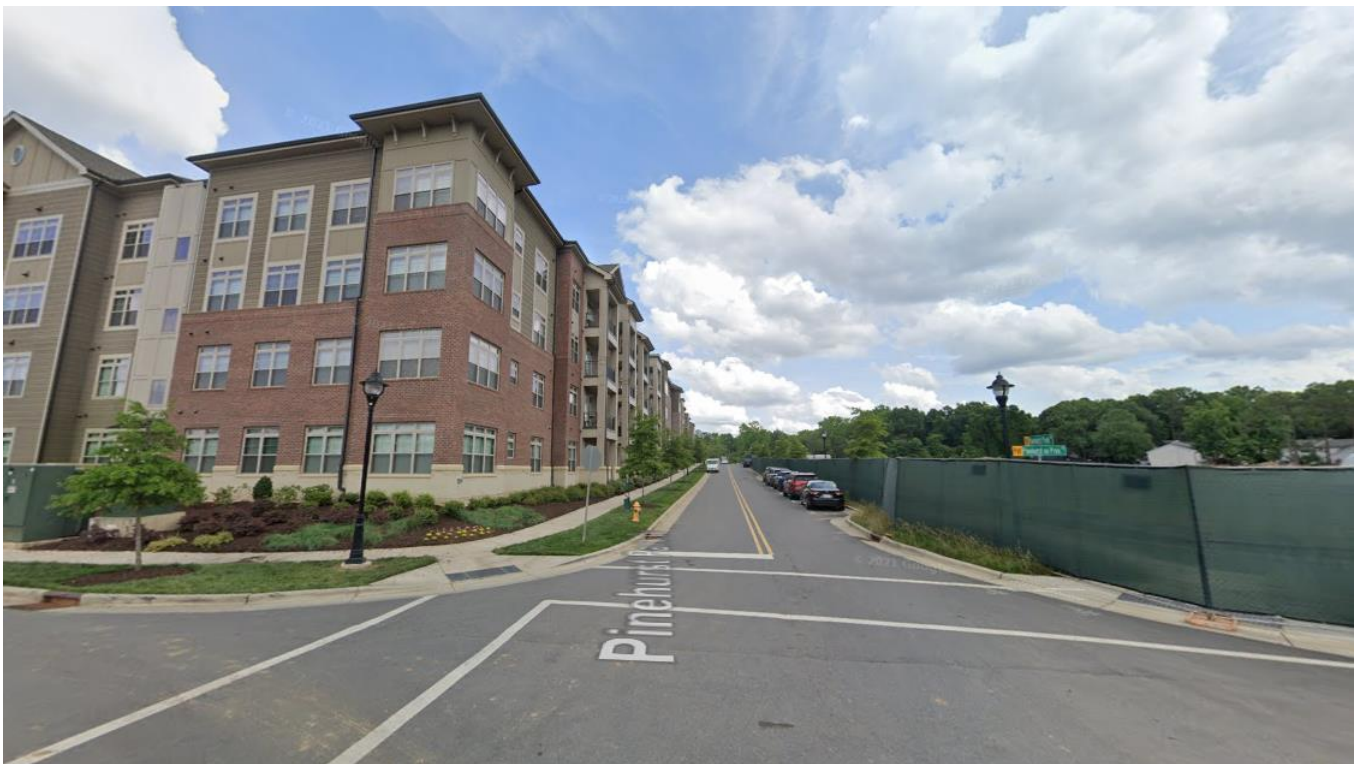
View of the site looking south from the intersection of Pinehurst on Providence Drive and Pinehurst Parkway. Building 3 in existing phase of the development is at the left of the image and Building 6 of the existing phase of the development is under construction at the right of the image.
