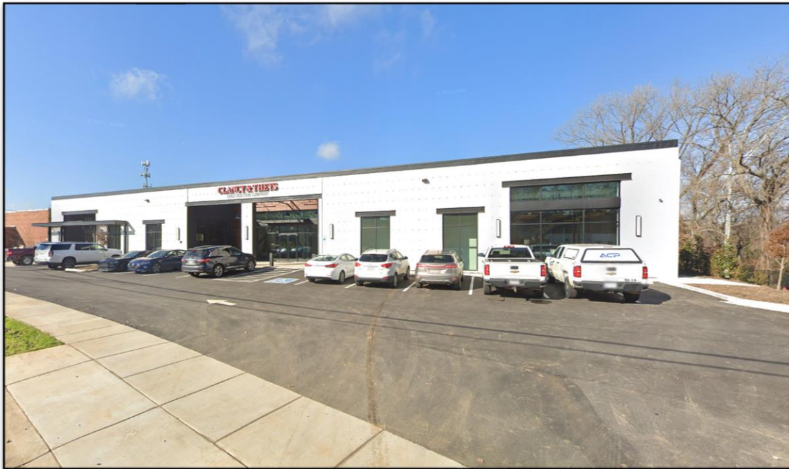
The requested rezoning sites are in one building, with the site spaces being at opposite ends of each other.
