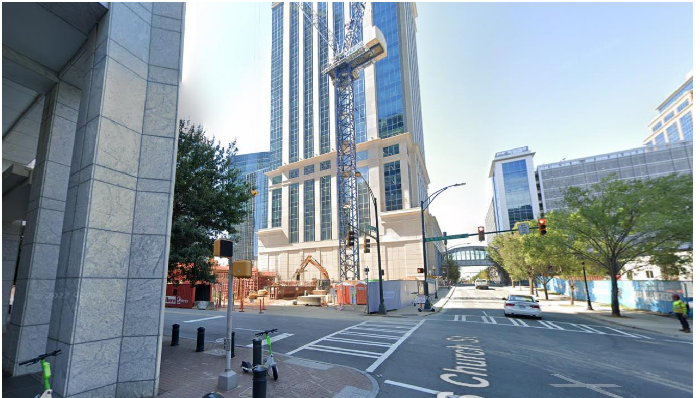
View of the site looking south from the intersection of South Church Street and East Brooklyn Village Avenue. The sign is proposed to be located on the building under construction at the southeast corner of this intersection.
