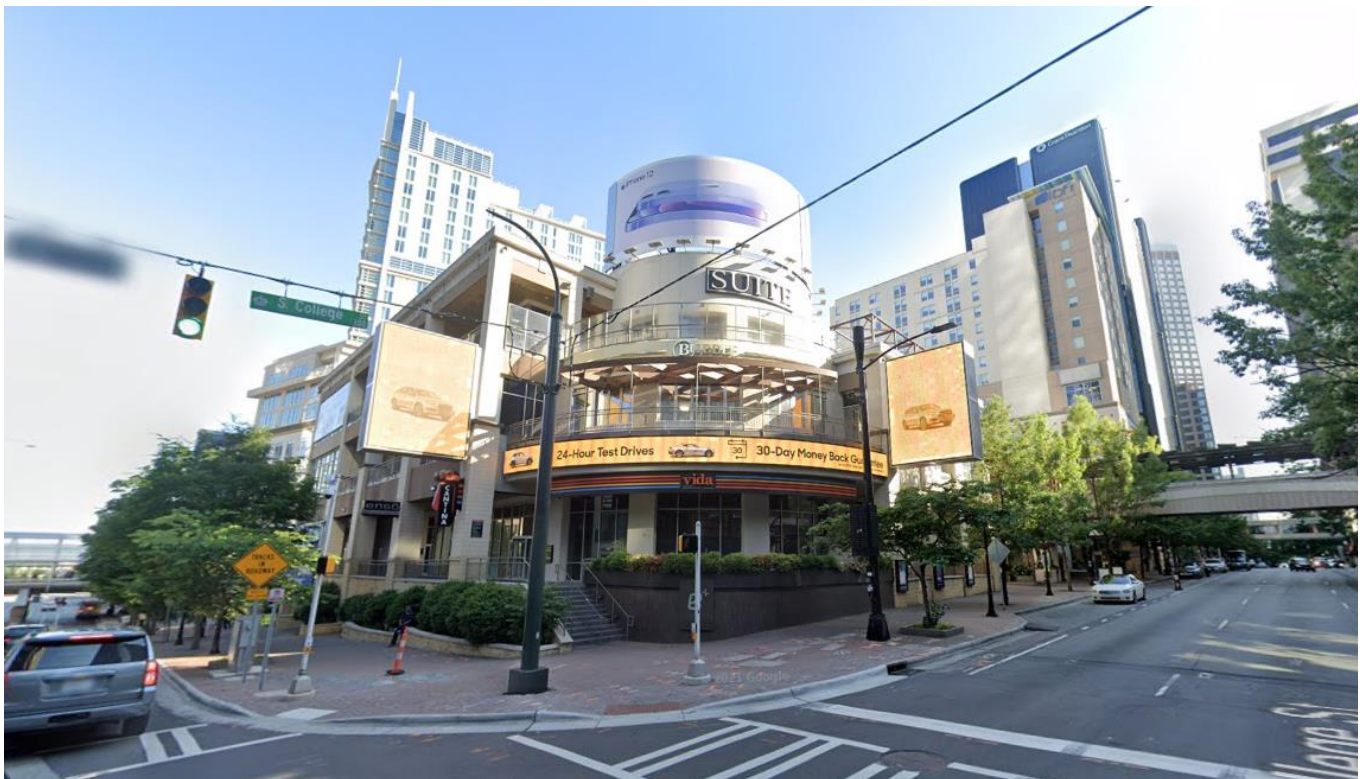
View of the electronic changeable copy wall and projecting signs located on Queen City Quarter. The projecting signs are approximately 234 square feet per sign face and the electronic banner sign is approximately 276 square feet. These signs were approved in 2013 by an administrative amendment to rezoning petition 2004-028.
