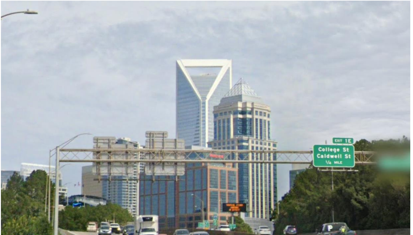
View of the tower looking east from I-277 on the inner loop of John Belk Freeway. The skyline sign is proposed to be mounted on the white upper horizontal portion of the building.
