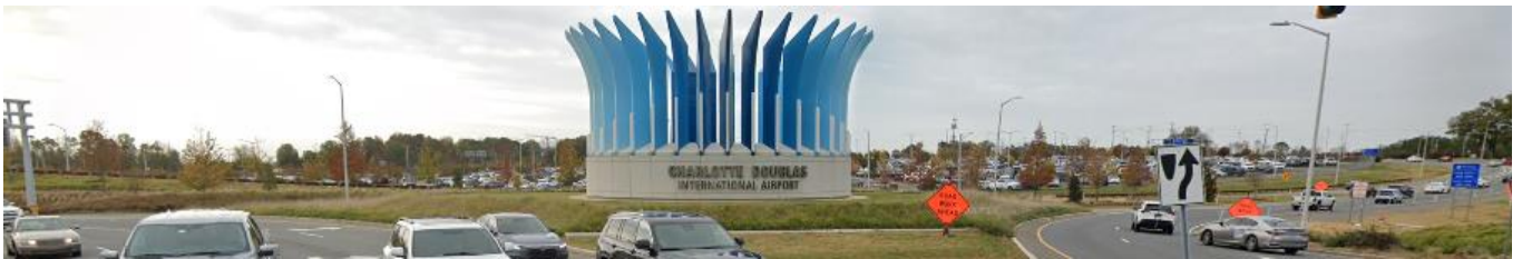
Street view of parking lots associated with Charlotte Douglas International Airport to the south of the site across Wilkinson Boulevard.
