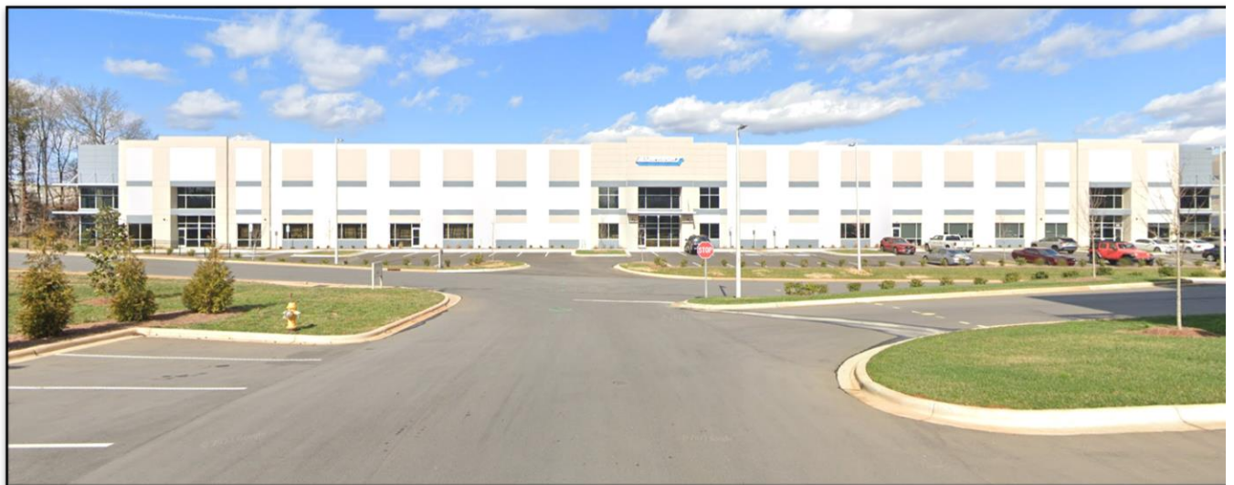
The site currently has an industrial use on the parcel.
