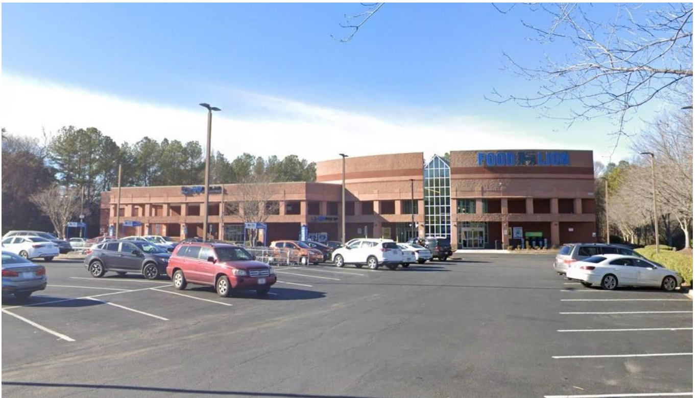
View of the Food Lion located just to the east of the site in a shopping center at the corner of Mallard Creek Road and West WT Harris Boulevard.
