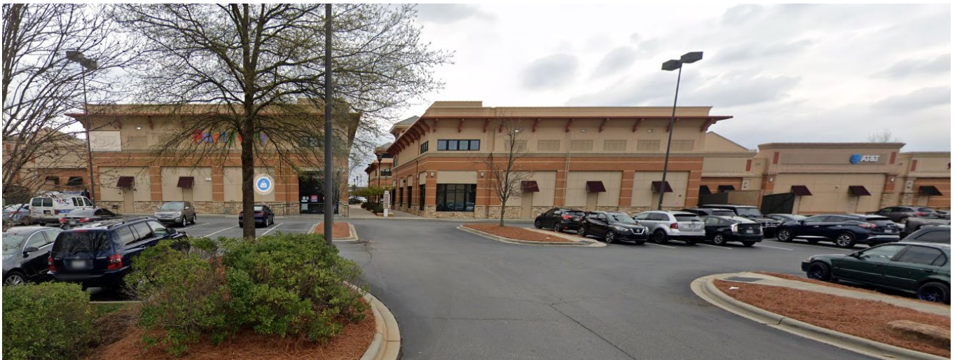
The property to the west along Northlake Commons Boulevard is Northlake Commons shopping Center.
