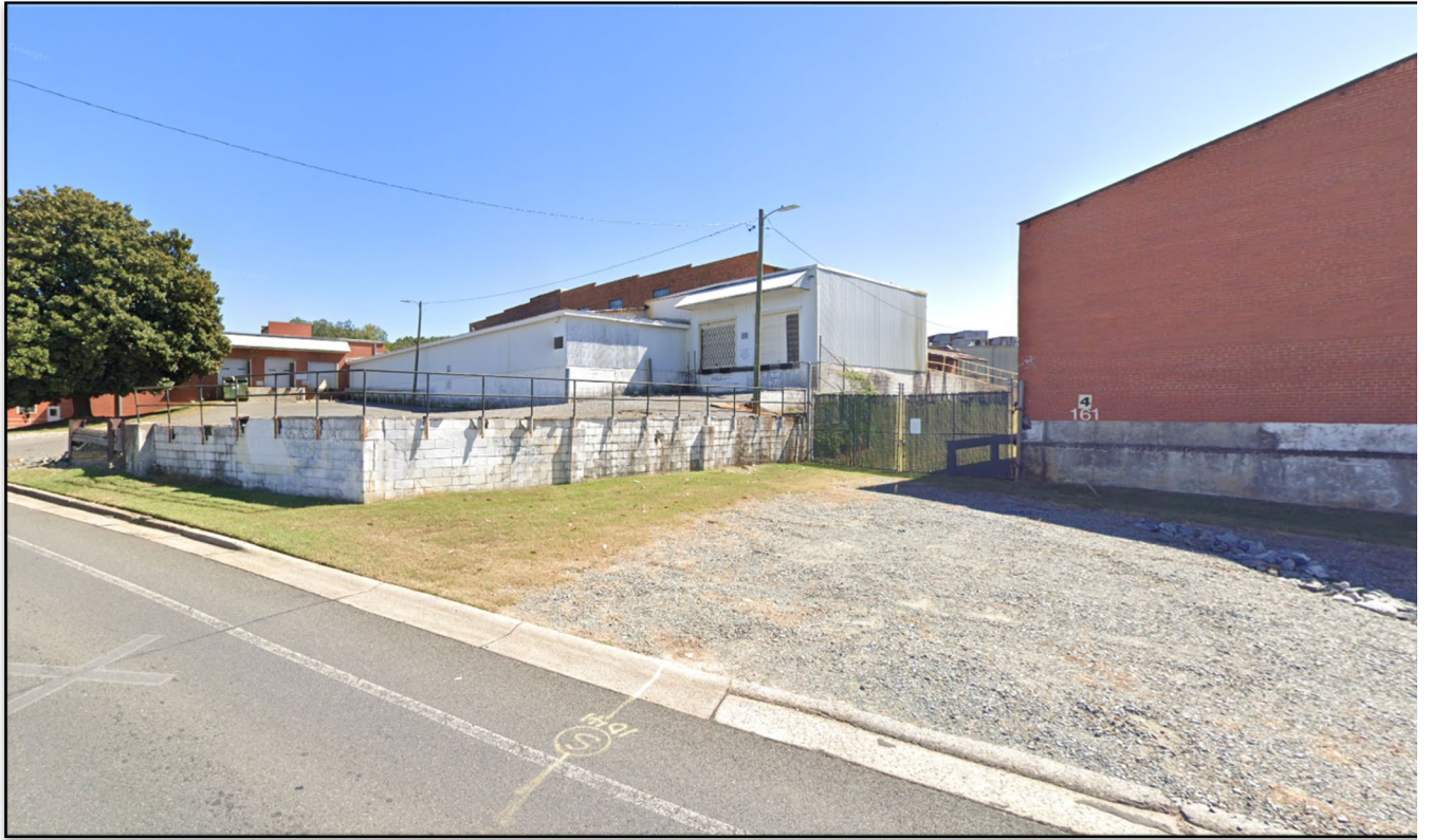
East of the site is a large manufacturing building.
