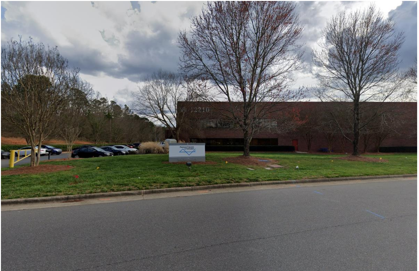
South of the site is a office/industrial building.
