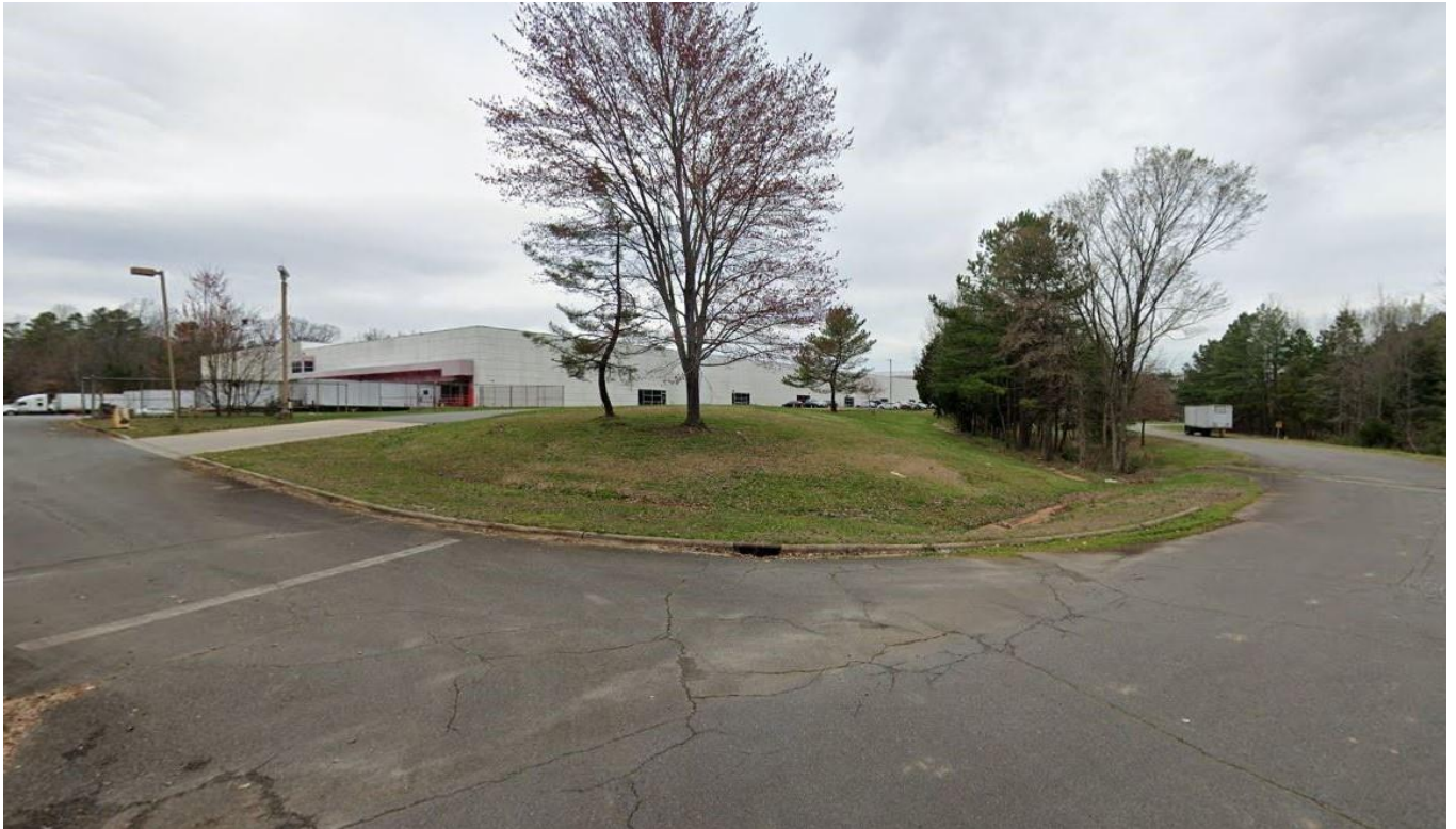
View of the site looking north from the Morris Estate Drive. The property is currently developed with a light manufacturing, assembly, and warehousing facility.
