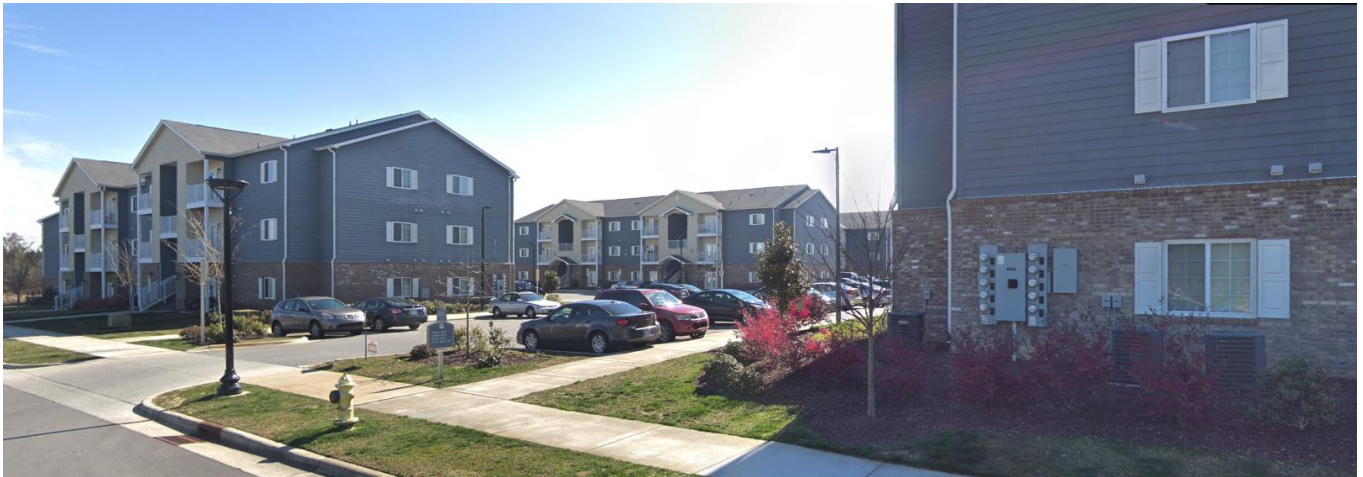
The property to the northwest along Grafton Regis Lane is developed with multi-family apartments.
